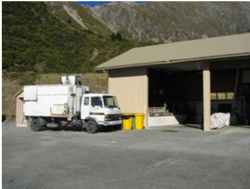
Figure 15 – Existing solid-waste truck and workshop facility
