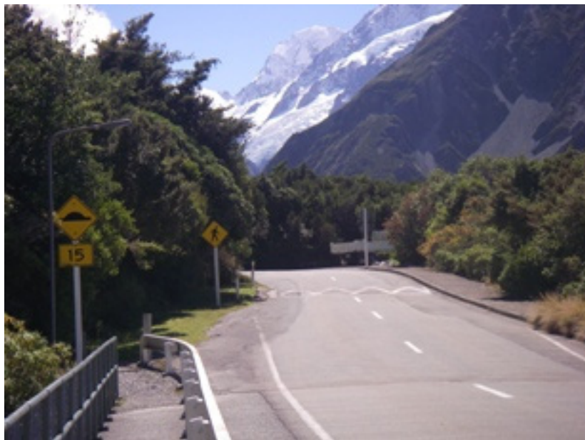
Figure 17 – Village loop road (Bowen Drive)
