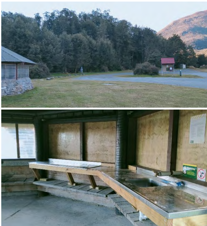
Figure 55: The current Klondyke Corner Camping Ground & Kitchen Facility
