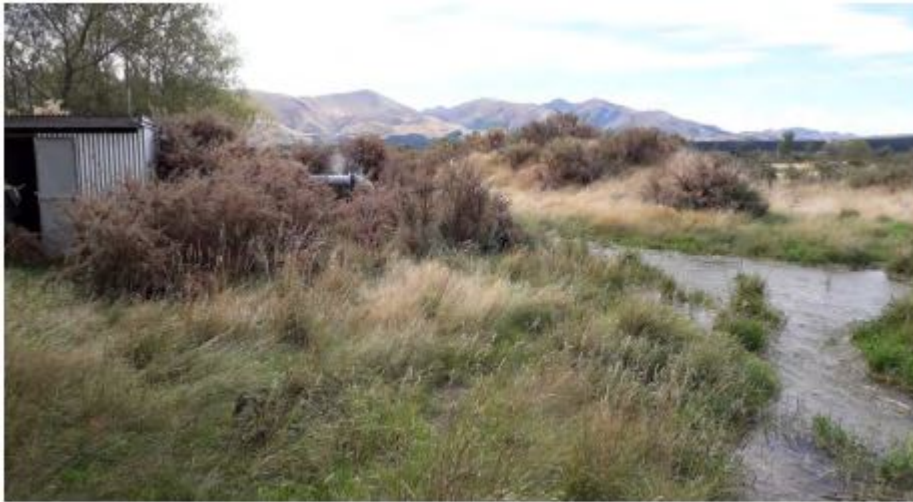
Photo 3: Looking west at the existing irrigation channel and pump station (existing Hassall easement 47898-OTH)
