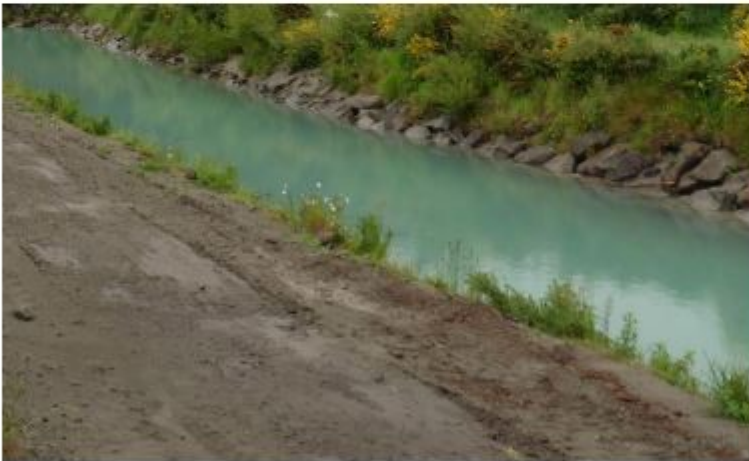
21. This is a typical bywash or fish bypass race, (utilising in situ riverbed gravels without rock rip rap armouring).
