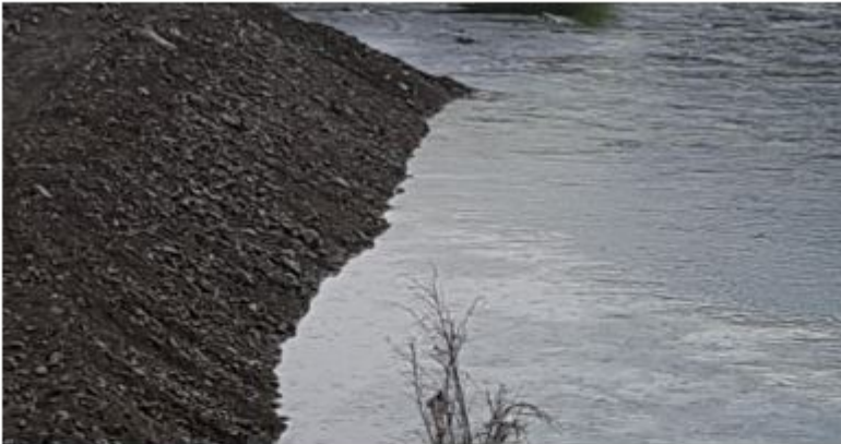
20. Rip rap rock may be required to line this slope. An example is shown below.
