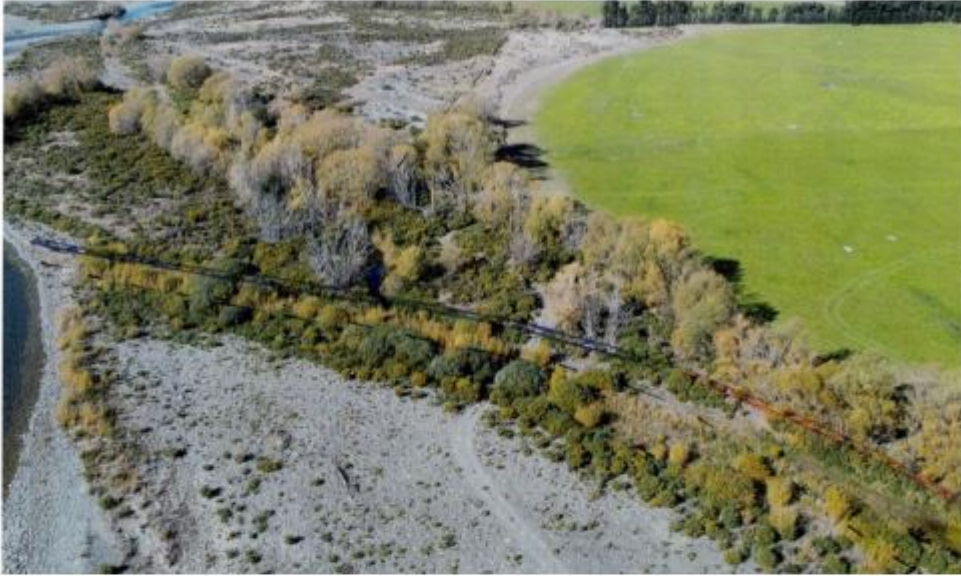
13. The flood protection works encroach on the marginal strip in the area circled in red on the below photo.
