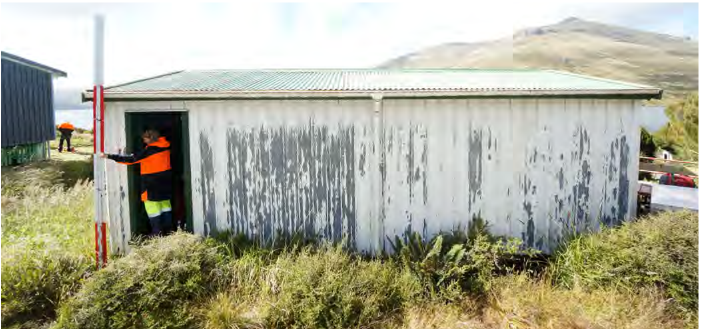
Figure N3 BELOW Elevation to the west, from the main walkway. The cladding to this elevation has been replaced,
