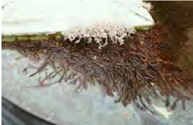
Figure J1 ABOVE Growth in and extending out of a water tank.
