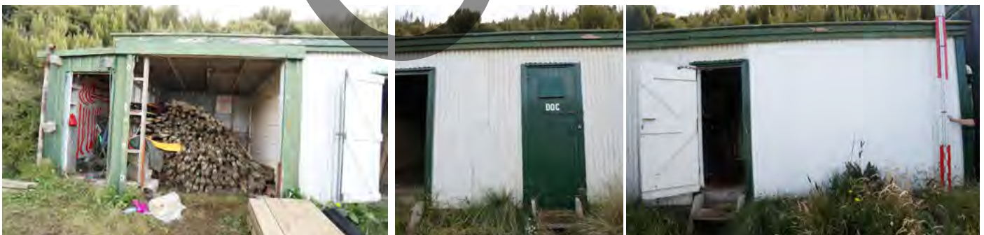
Figure L2 ; L3 ; L4 The east elevation of the Carpentry store on the far right, the vegetable store labelled "DOC" in the centre, and the building equipment and timber stores on the far left.
