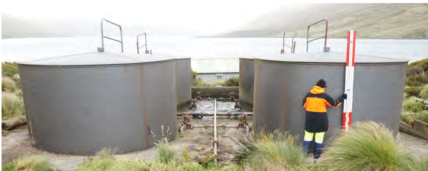
Figure X1 FAR TOP South elevation of the water tanks.
