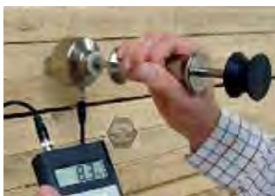
Figure 1-5 BELOW A sliding hammer was used to check moisture levels INSIDE the wall
