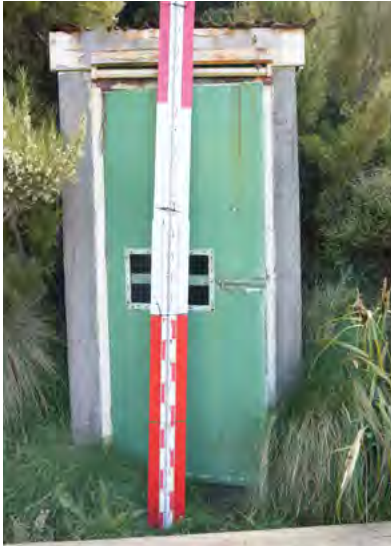
Figure L1 ABOVE The Meat hanging and butchery hanging room. The roof and walls are in very poor condition.
