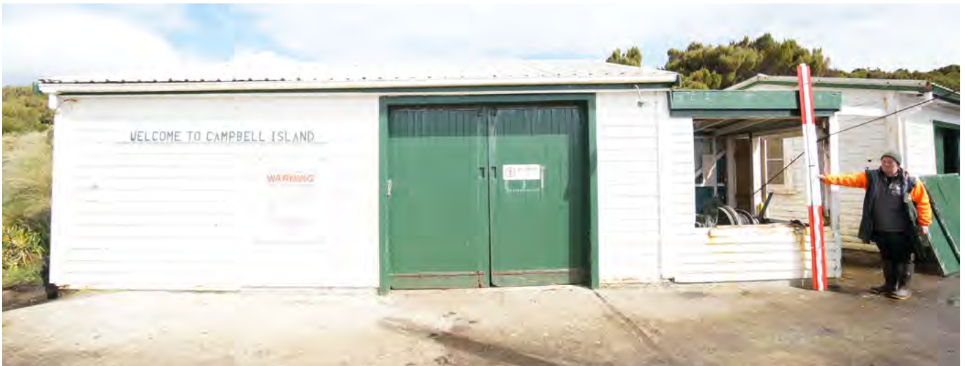
Figure S1 BELOW East elevation of Jetty Store with winch alcove, with window openings removed and on the ground leaning against the Spirits / Paint store.
