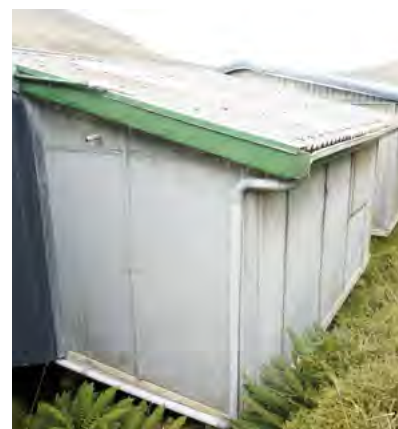
Figure G1 ABOVE Hostel sleeping annex. West elevation.
