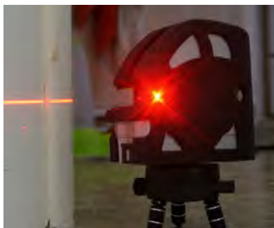
Figure 1-4 ABOVE An industrial laser was used to check the condition of the foundations, these measurements are on the plans, eg FFL +10.
