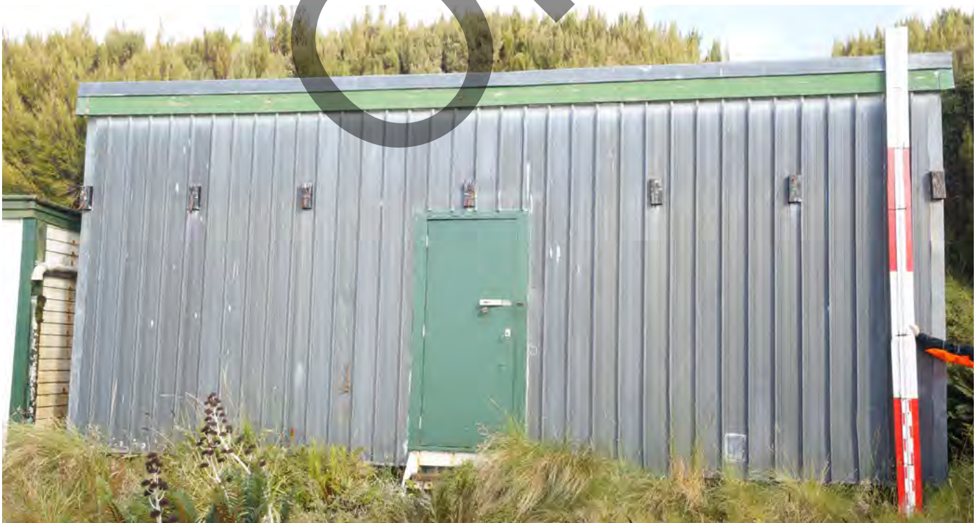
Figure J1 BELOW The east elevation of the Cool Store.
