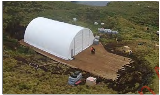
Figure 19: Temporary helicopter hangar, Antipodes Island 2016
