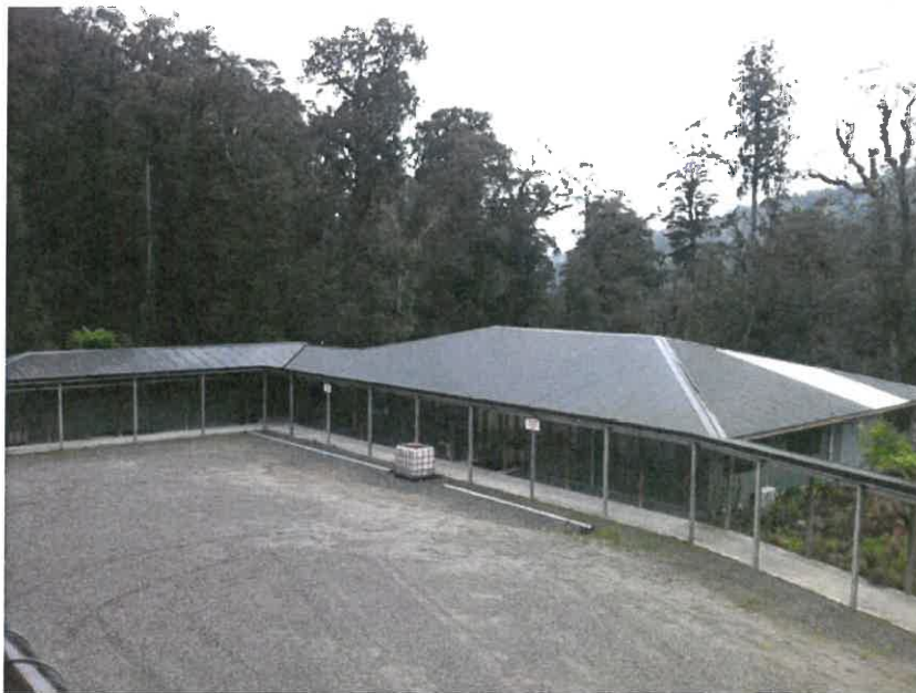
Amenity buildings Pike River Mine
