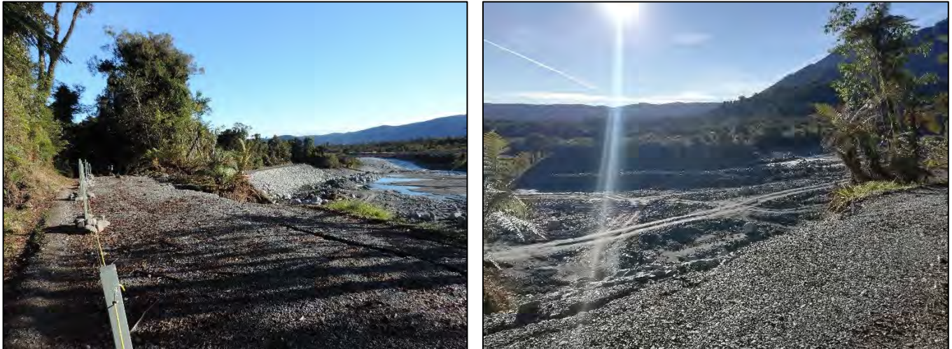
Figure 1-8 – Photos of the South Washout 1 location – looking downstream & across
