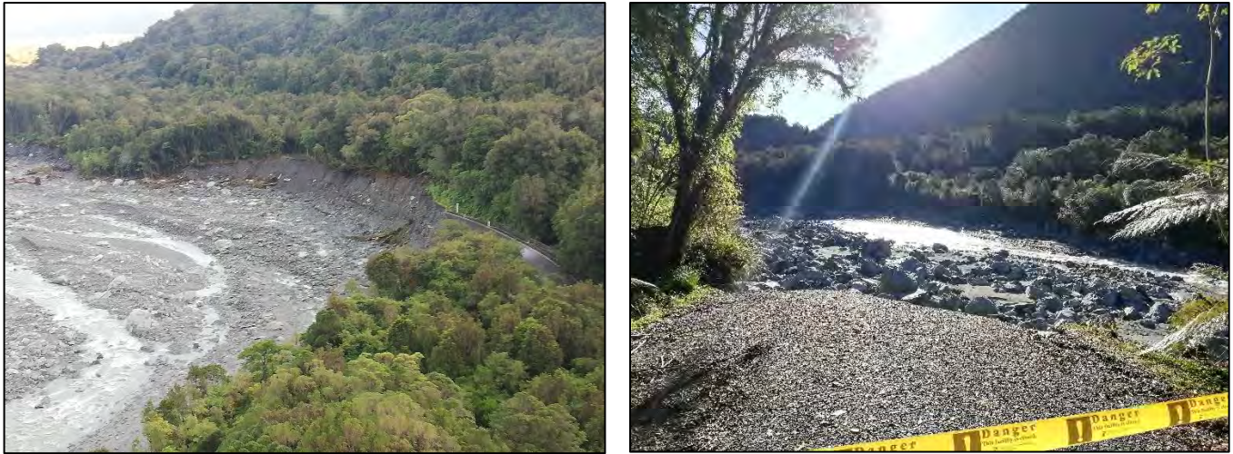
Figure 1-10 – Photos of the South Washout 3 location – looking upstream & downstream
