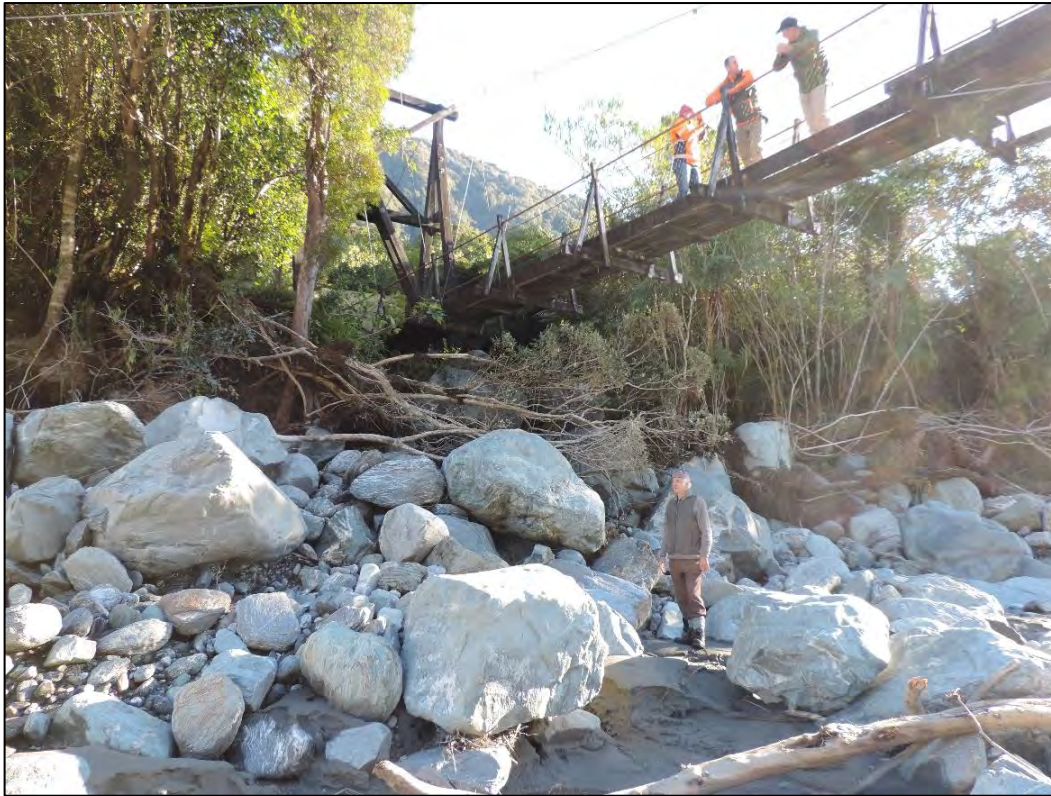
Photo 17 - The left (south) side of the bridge, showing the large boulders that are stacked on this side of the river channel.
