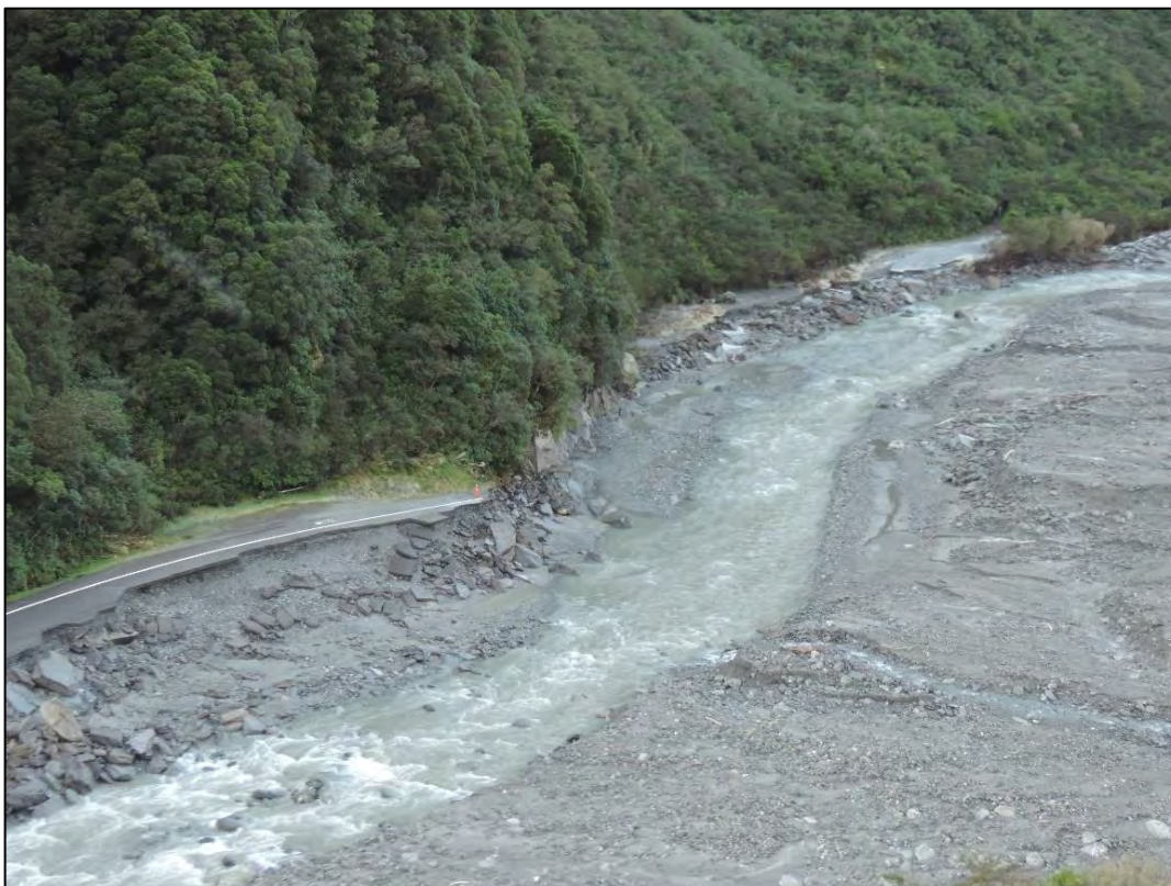
Photo 22 - North Washout 3 looking upstream. The bluff at the outer edge of the high mountains is the point between the two washouts, where the remaining seal ends.
