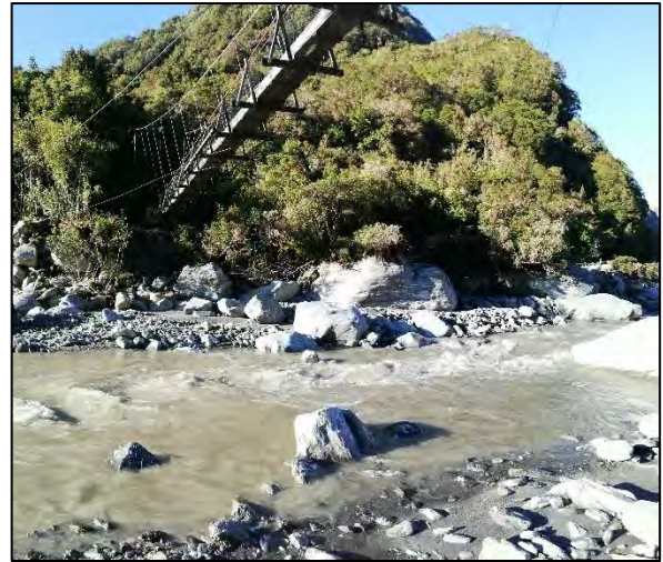
Figure 3-2 – True right bridge abutment protected by boulders. Left abutment exposed and vulnerable
