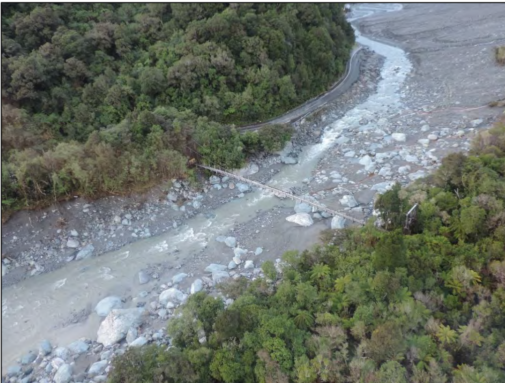
Photo 14 - Looking upstream over the footbridge, showing the bottom edge of the Mills Creek fan just above it. North Washout 2 is also just above the footbridge, with the Fox River now squeezed between the fan and the roadway.
