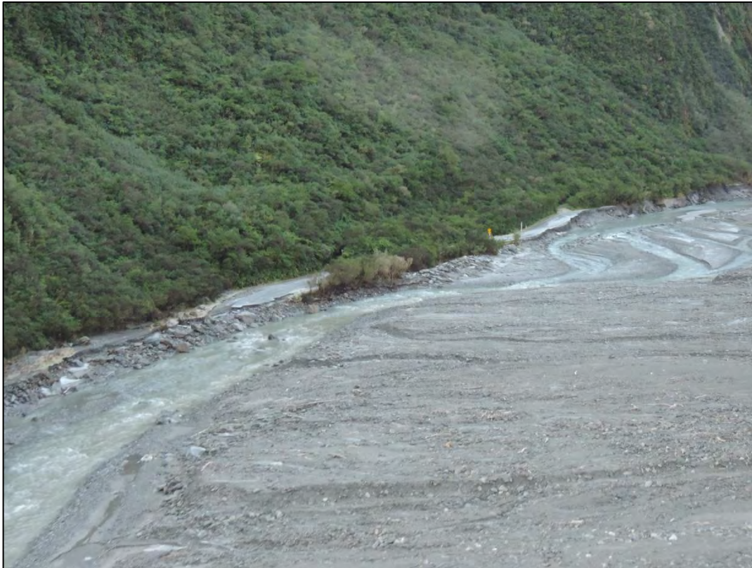
Photo 23 - North Washout 3 and upstream, showing the Fox River between the toe of the Mills Creek fan and the roadway along the edge of the very steep mountainsides.
