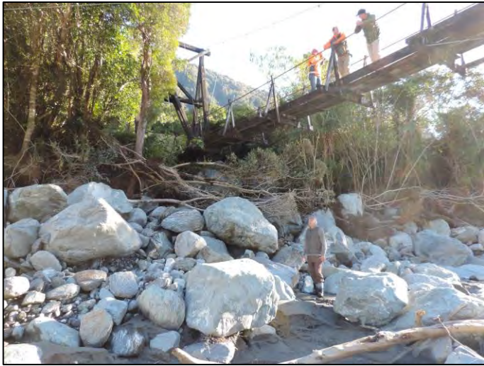
Figure 3-2 – True right bridge abutment protected by boulders. Left abutment exposed and vulnerable
