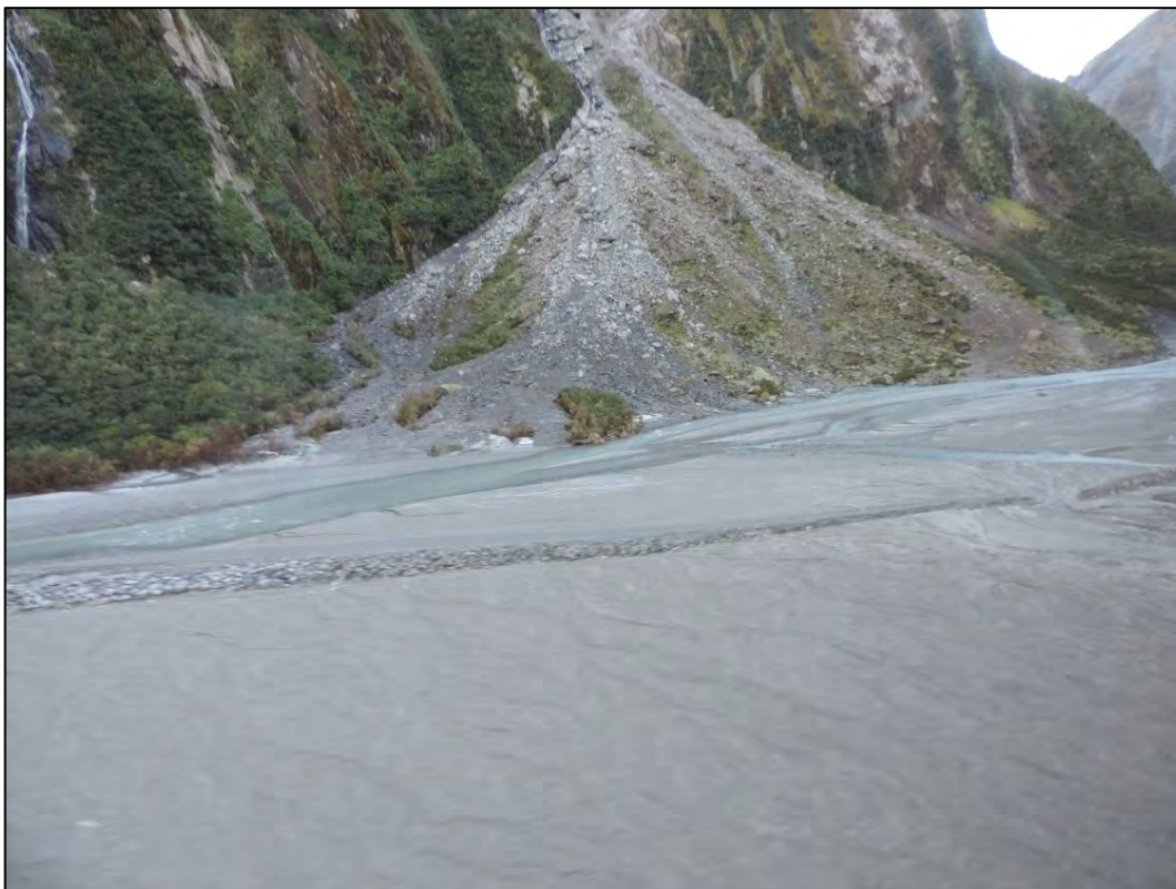
Photo 18 - The Undercite fan on the right (north) side, which is still active. The road was re-aligned into the river bed to go around this fan after it first formed.
