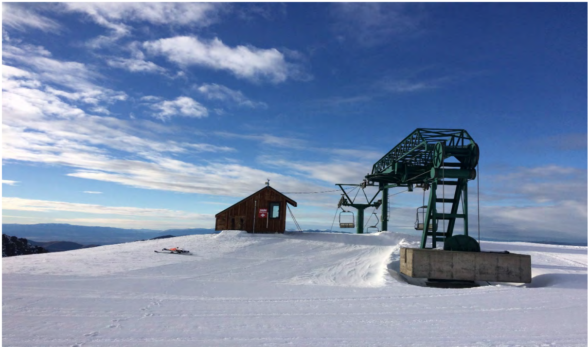
Figure 2: Existing return terminal and “Top Shack”.
