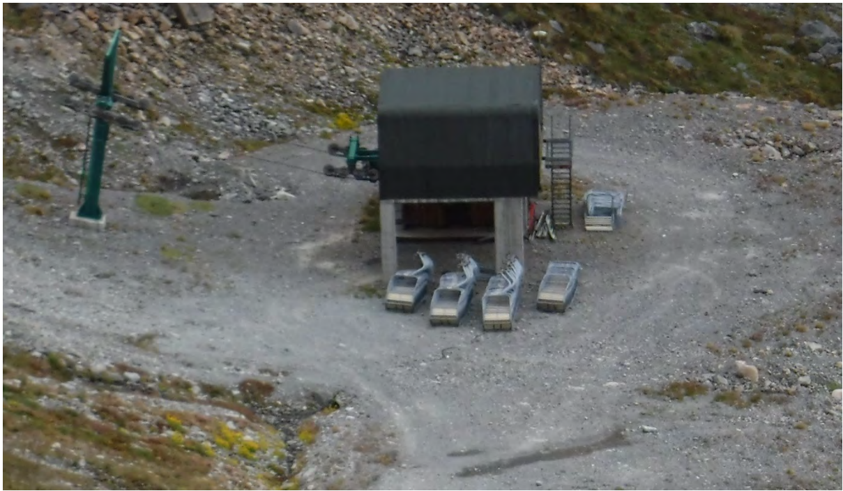
Figure 1: Existing drive station and base building.
