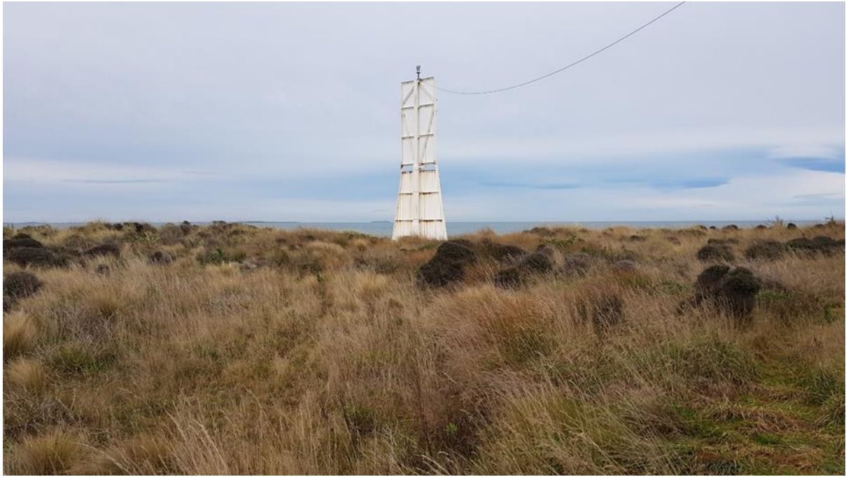
Figure 5-Proposed location looking from dirt road
