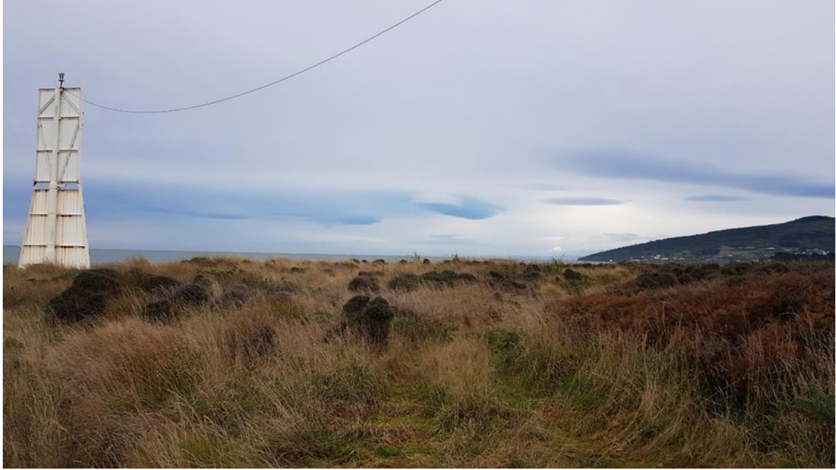
Figure 3-Looking from gravel road down dirt track towards lead light
