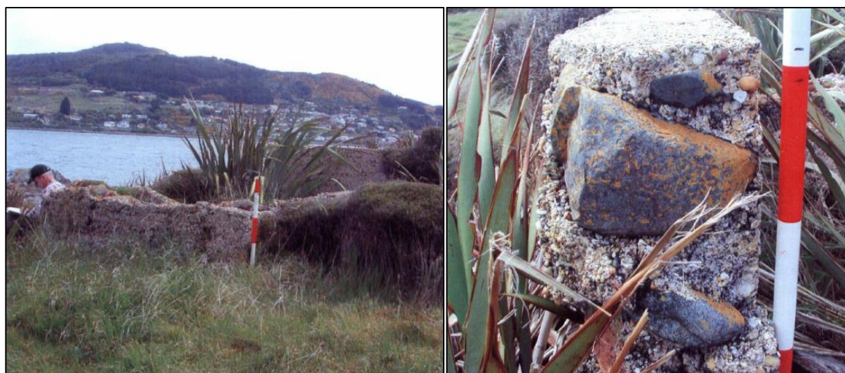
Figure 6-2 Photo of concrete structure at E47/169 (ArchSite).
