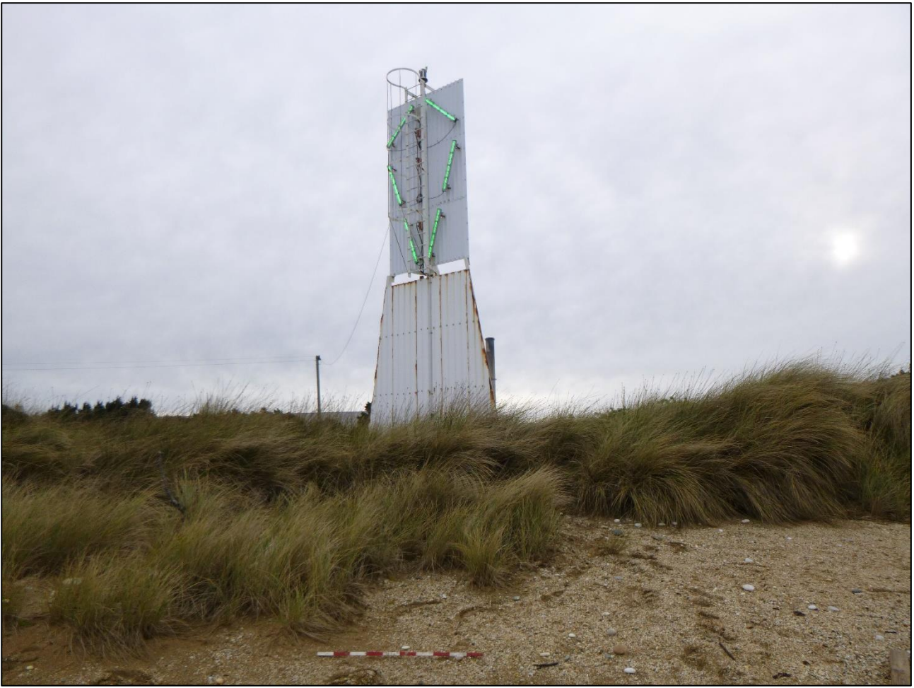
Figure 7-4 View of the extant beacon at Beacon 1 from the beach (looking north). Note existing overhead power lines, to be replaced with the solar system.
