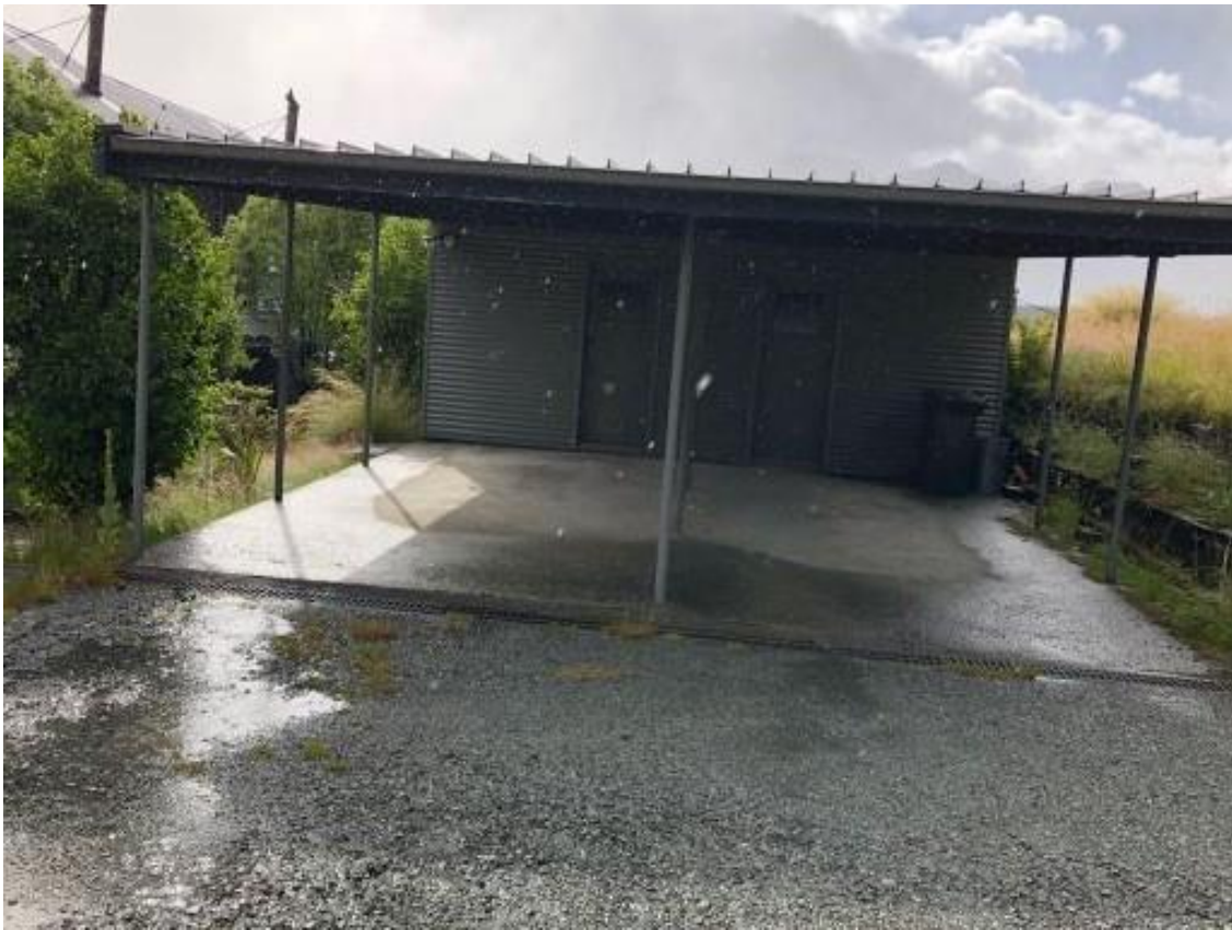
Photo of carport (partial view)
