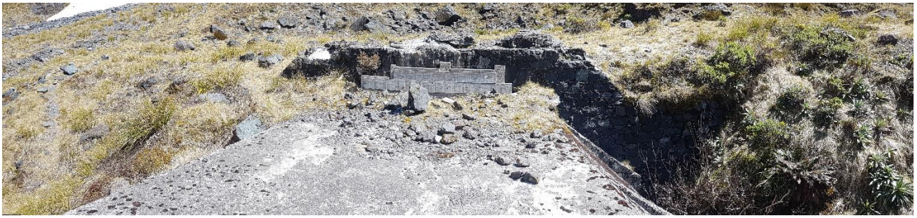
Photo 7: Homer Tunnel Eastern Portal original stacked rock wall and surrounding vegetation.
