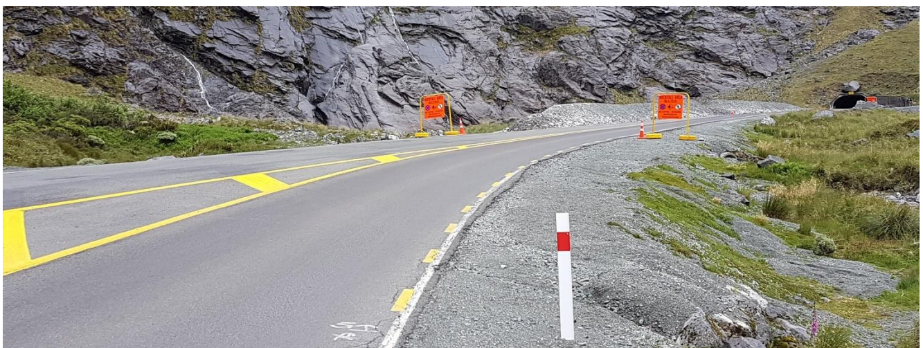
Photo 13: SH94 200m east of Homer Tunnel eastern portal (at traffic light stop lane location).
