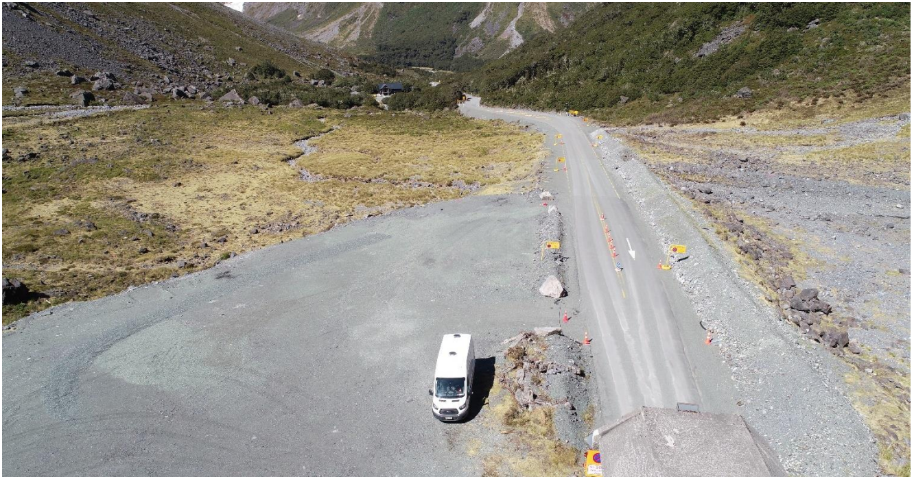
Photo 2: view east from above Homer Tunnel Eastern portal along SH94.
