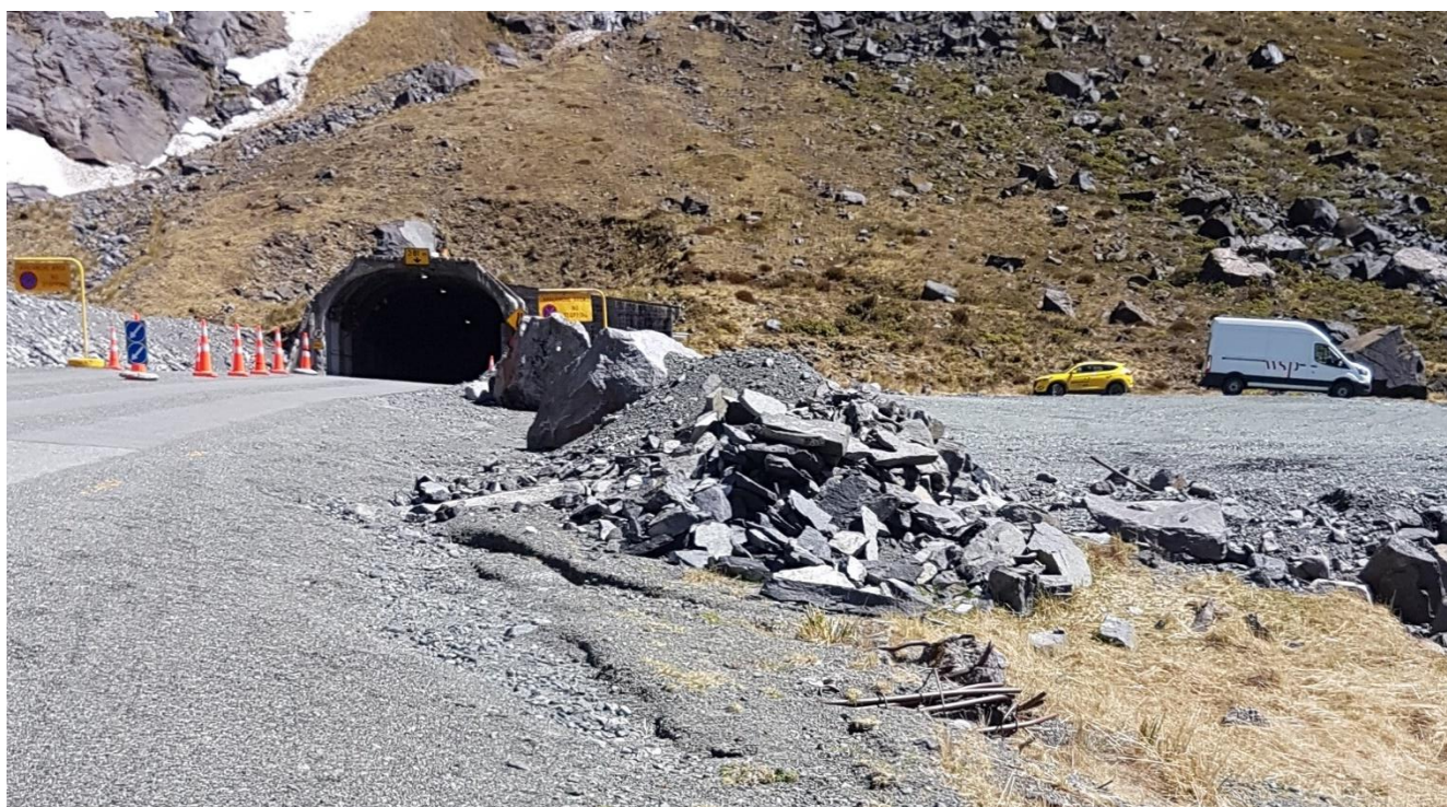
Photo 6: view west along SH94 to avalanche shelter remains.
