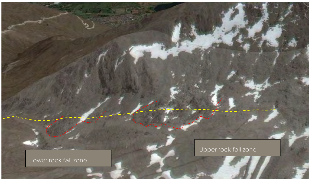
Figure 6-1: Lift Line and rock fall debris fans
