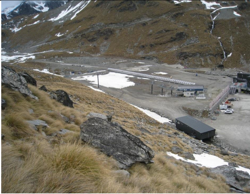
Figure 9: Looking down towards base building and location of proposed bottom station/terminal in carpark behind medical building (to be relocated) (Photo 055)
