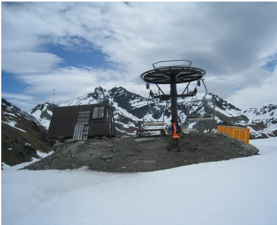
Figure 14: Top of Sugar Bowl chairlift and associated structures to be decommissioned (Photo 038)
