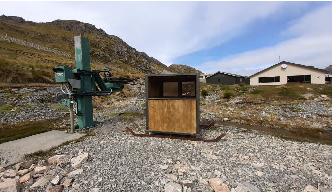
Figure 37: Platter lift hut and platter lift drive station
