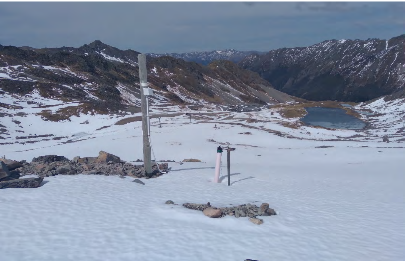
Figure 58: Hydrant with electric supply on post located above terrain park
