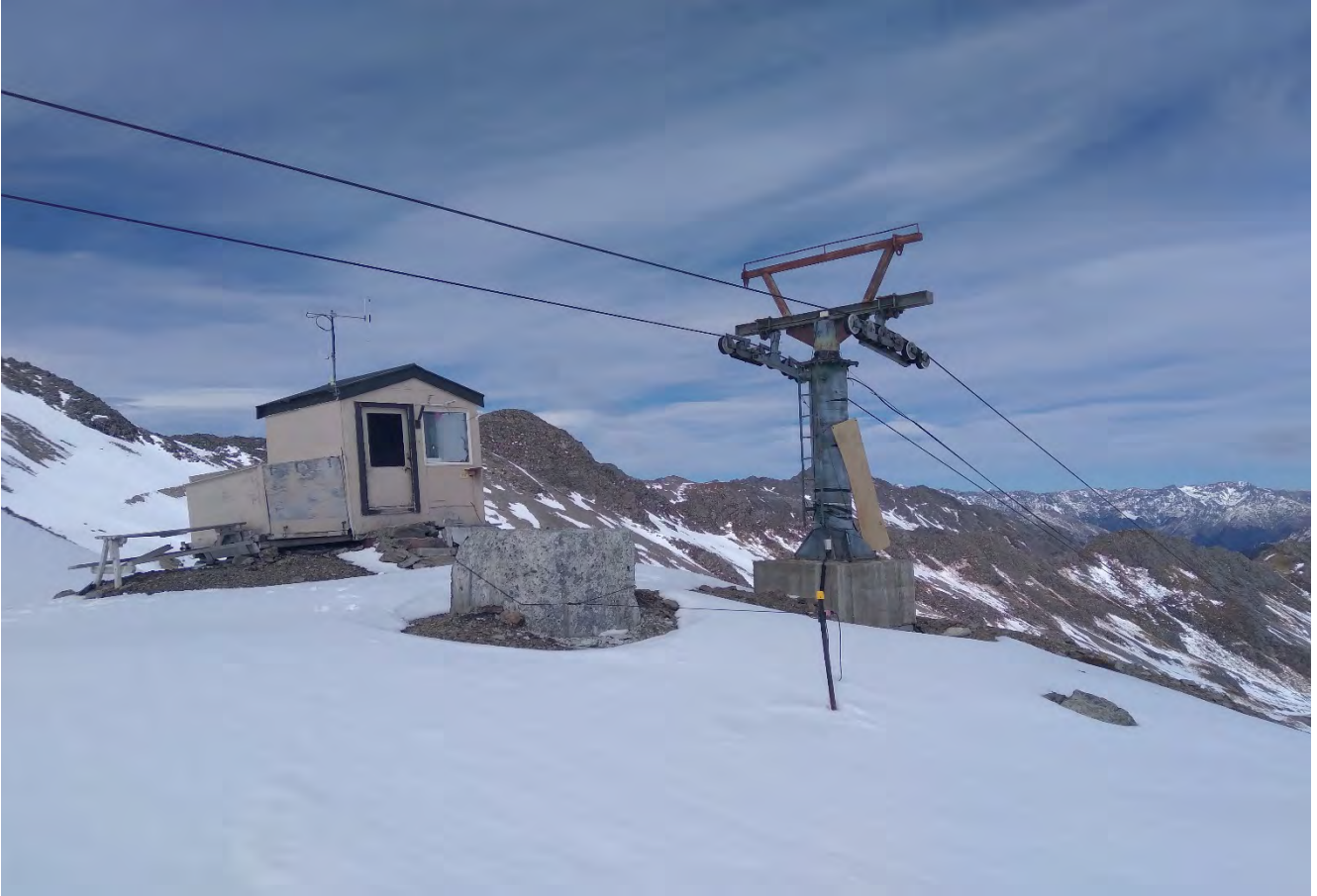
Figure 36: T-bar - top hut and tower 12
