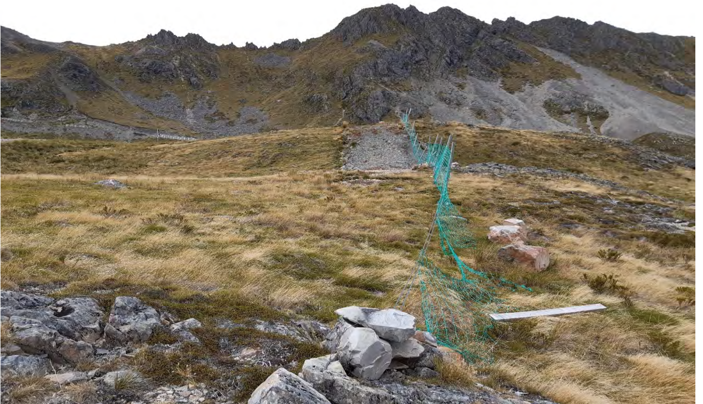
Figure 51: Tubing lift site with safety fence
