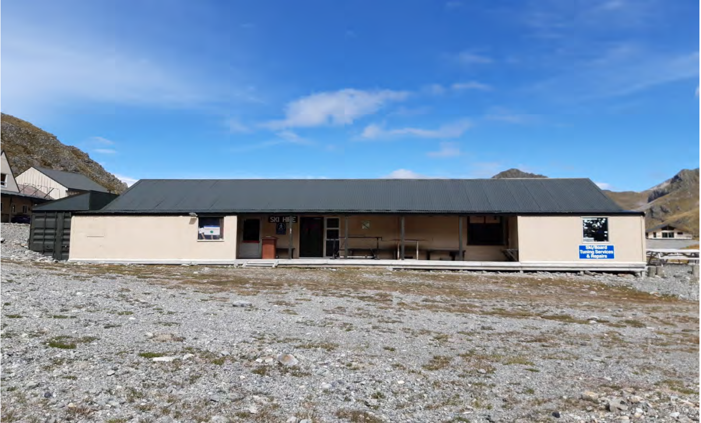
Figure 17: Ski hire and repair building with 100KVA generator shed at LH end of the building
