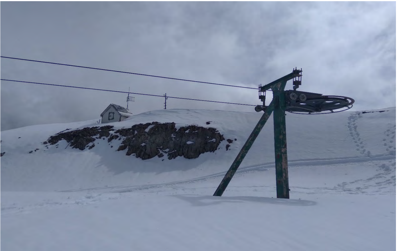
Figure 44: T-bar lift – return terminal
