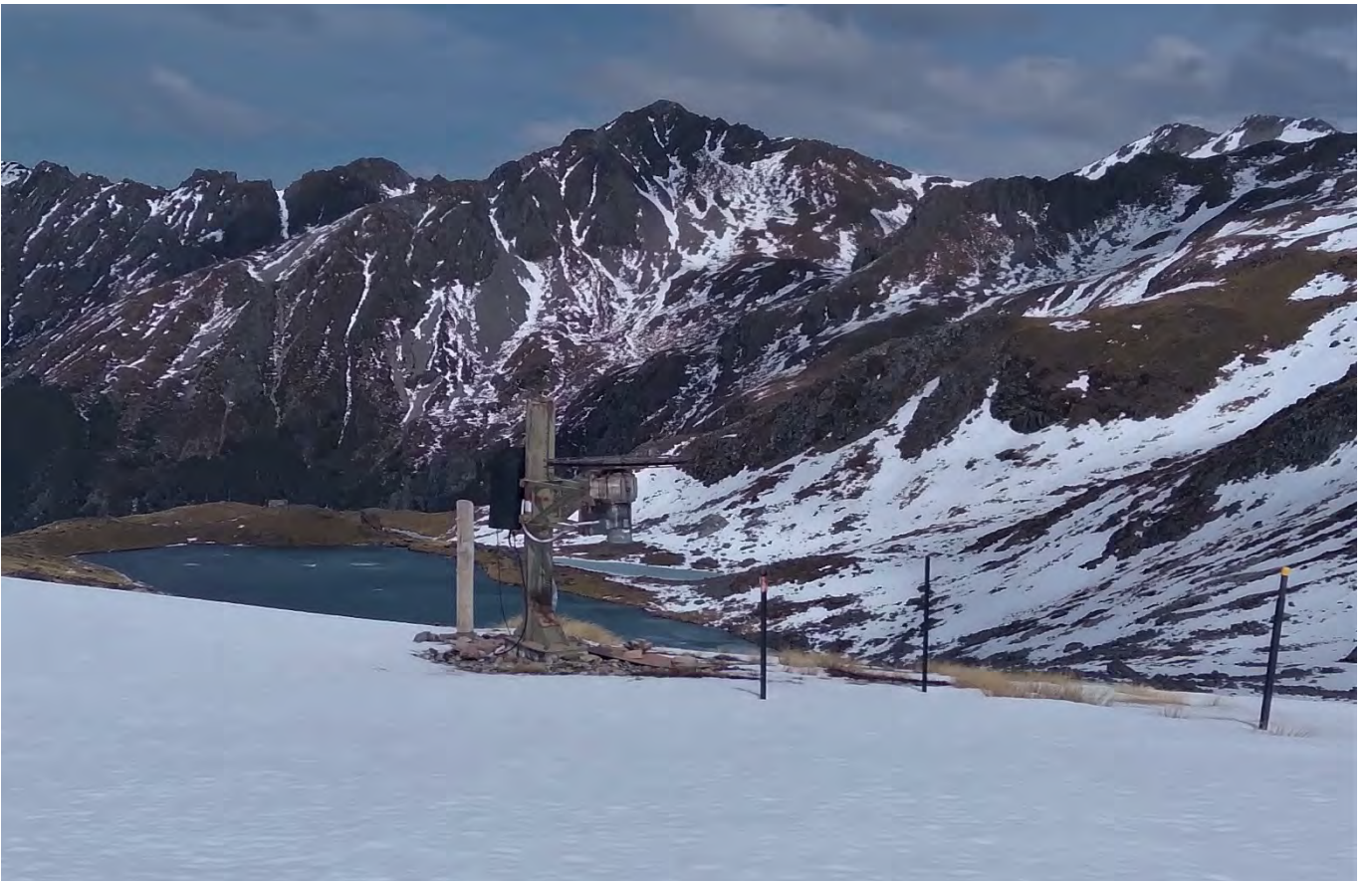
Figure 49: Terrain park lift drive terminal
