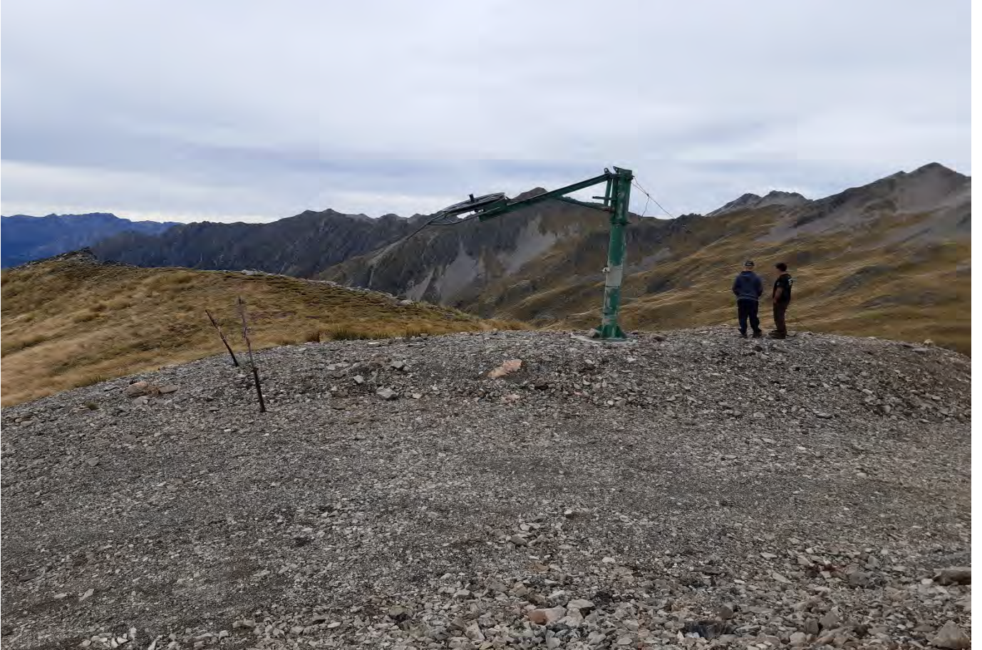
Figure 46: West bowl lift return tower at top of ridge
