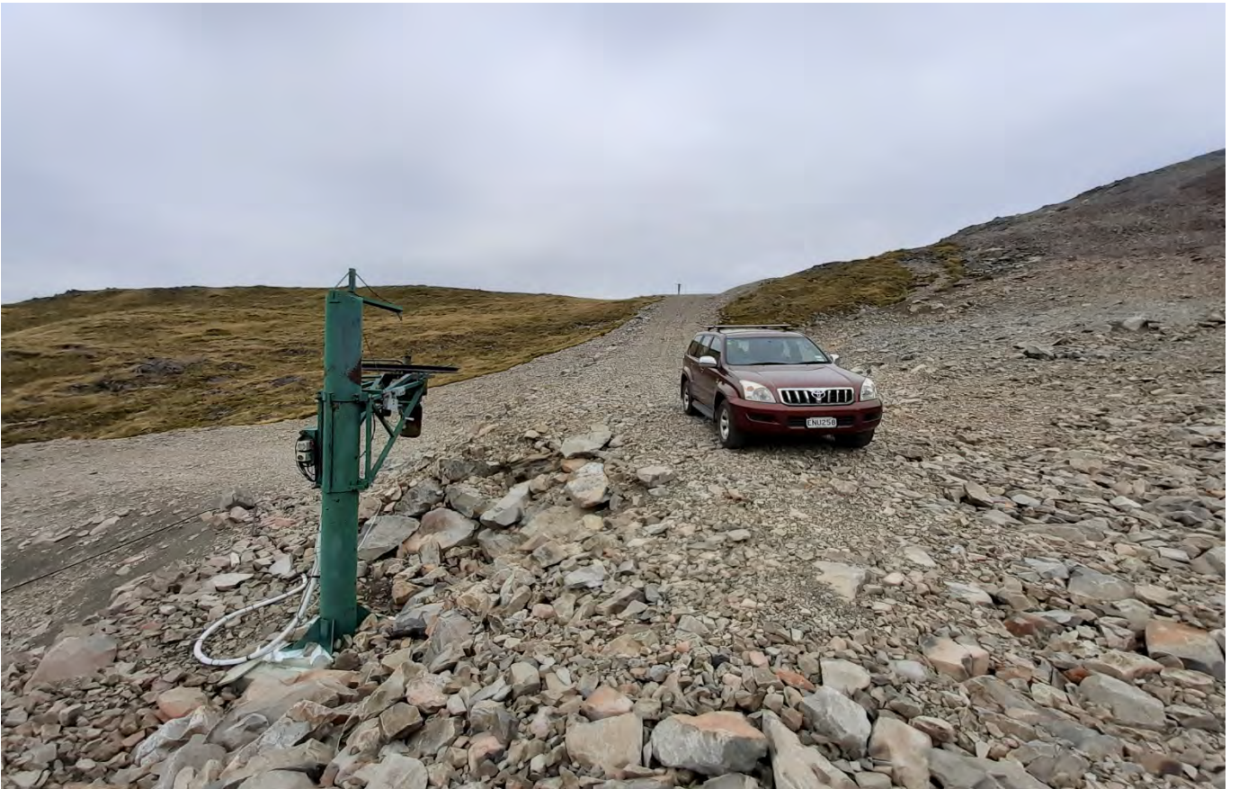
Figure 47: West Bowl drive terminal looking towards ridge
