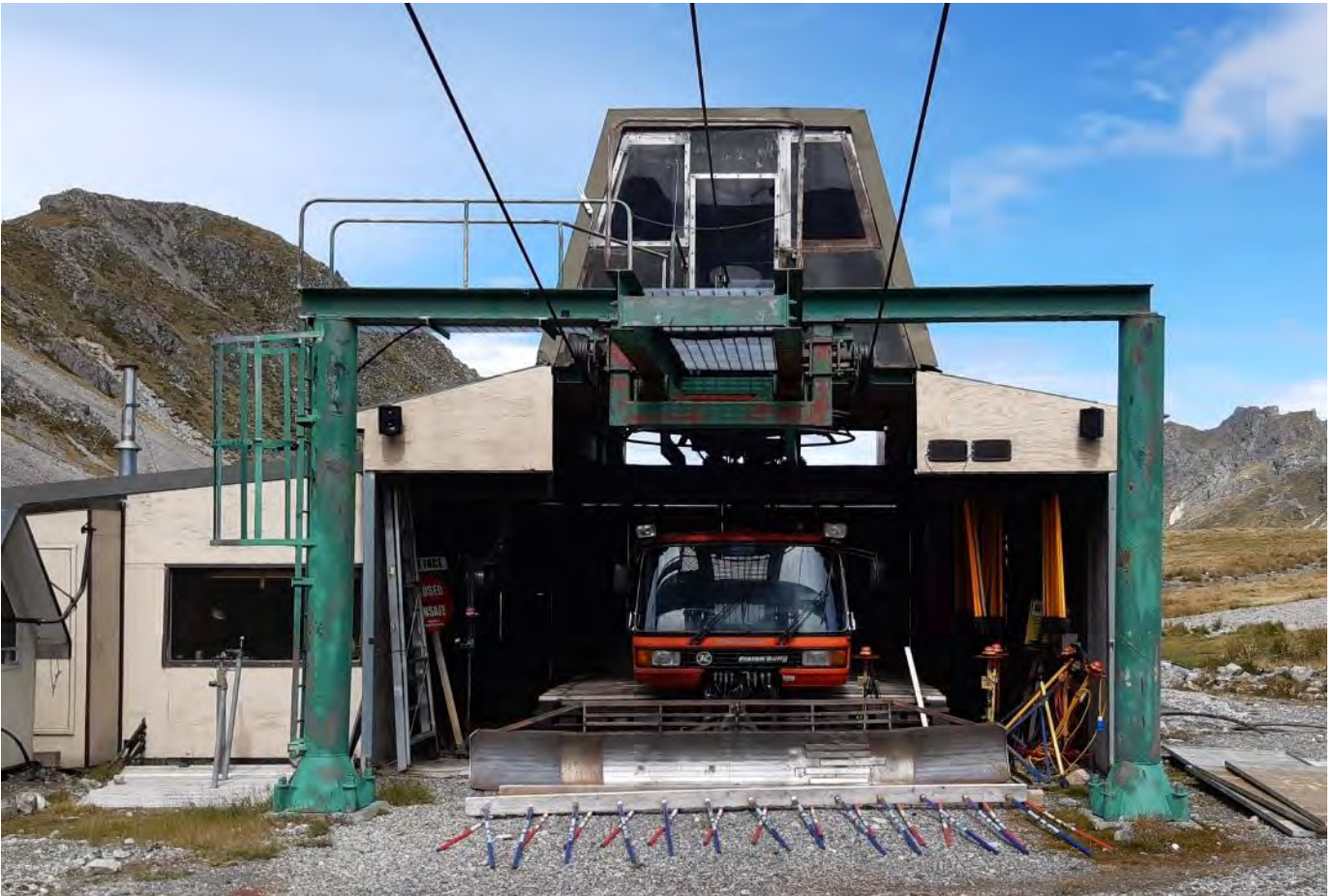
Figure 32: T-bar drive terminal
