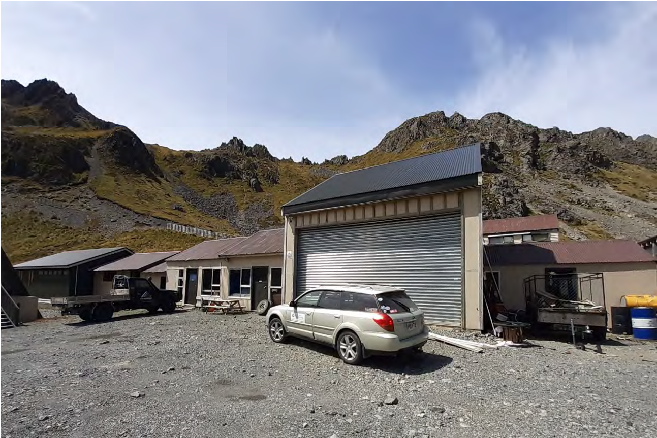
Figure 24: Workshop, staff room and staff accommodation
