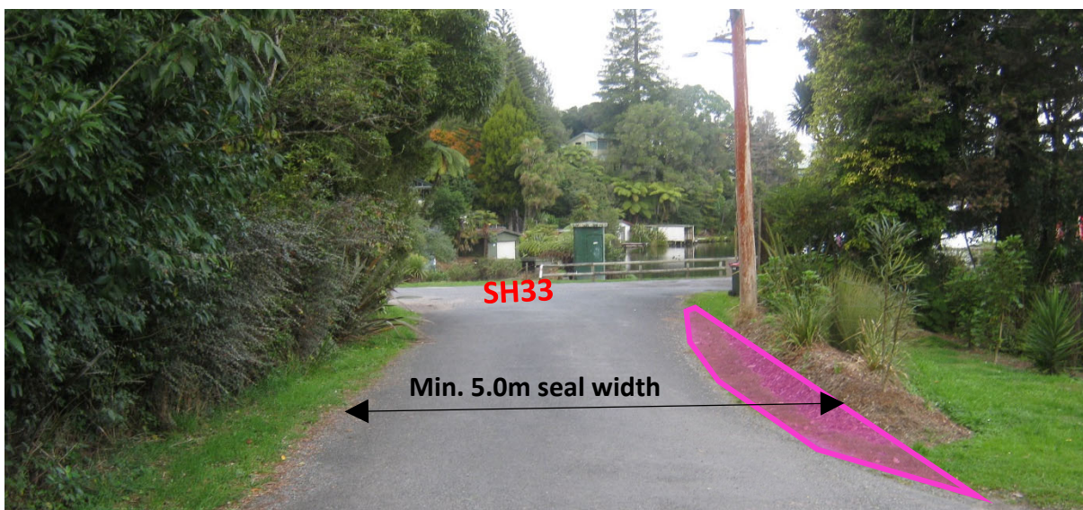
Figure 6: Proposed driveway seal widening
