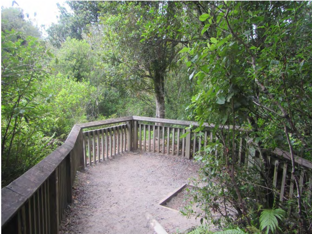
Plate 7: Existing track barrier near proposed location of Platforms 4 (right) and 5 (left). 10 January 2019.
