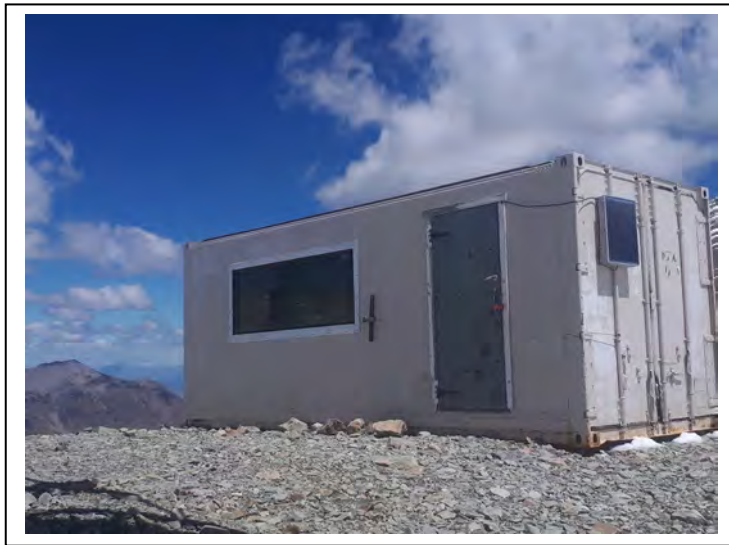
Figure 15 Top Chair Lift Operators hut
