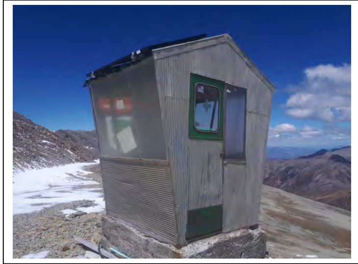
Figure 16 Top of the T Bar operators hut
