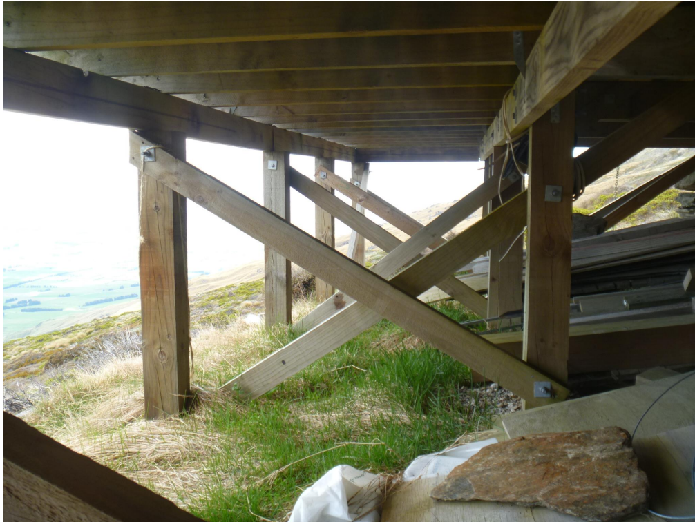
Photo 6 – Undeformed and well braced piles.
