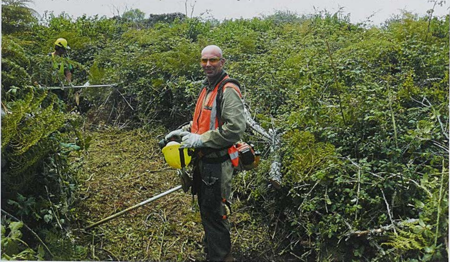
New sections of track on the Tauranga-Taupo River have had to be put through some pretty rough going. Rangers Ray Mond and Mike Hill are up to the task though. Photo by: Ray Packer
