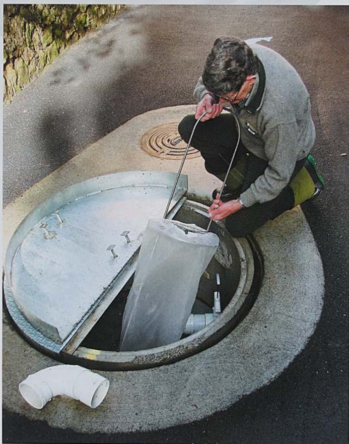
All of the outflow from the aquarium goes through a series of filters to ensure clean water is maintained and fish do not migrate to the surrounding ecosystem Photo by: Randal Hart
