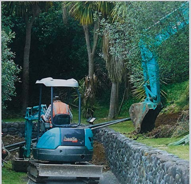
Installation of the rising main sewer pipe. Photo by John Webb.
