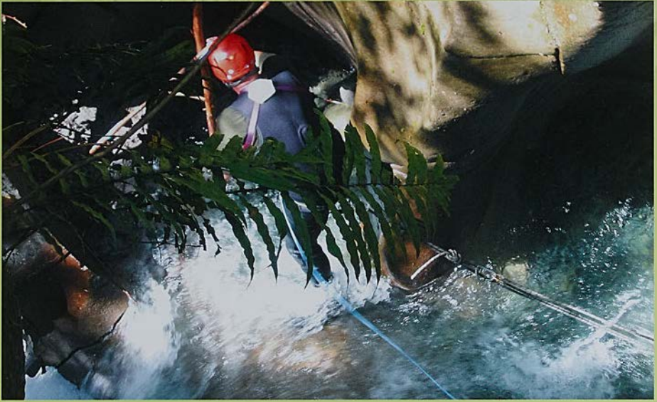
Not the place to be working without a harness and well anchored rope. Waioataka Gorge 2009.
