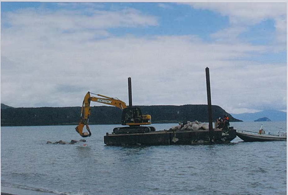
30 tonnes of rocks being placed onto the artificial reef.
