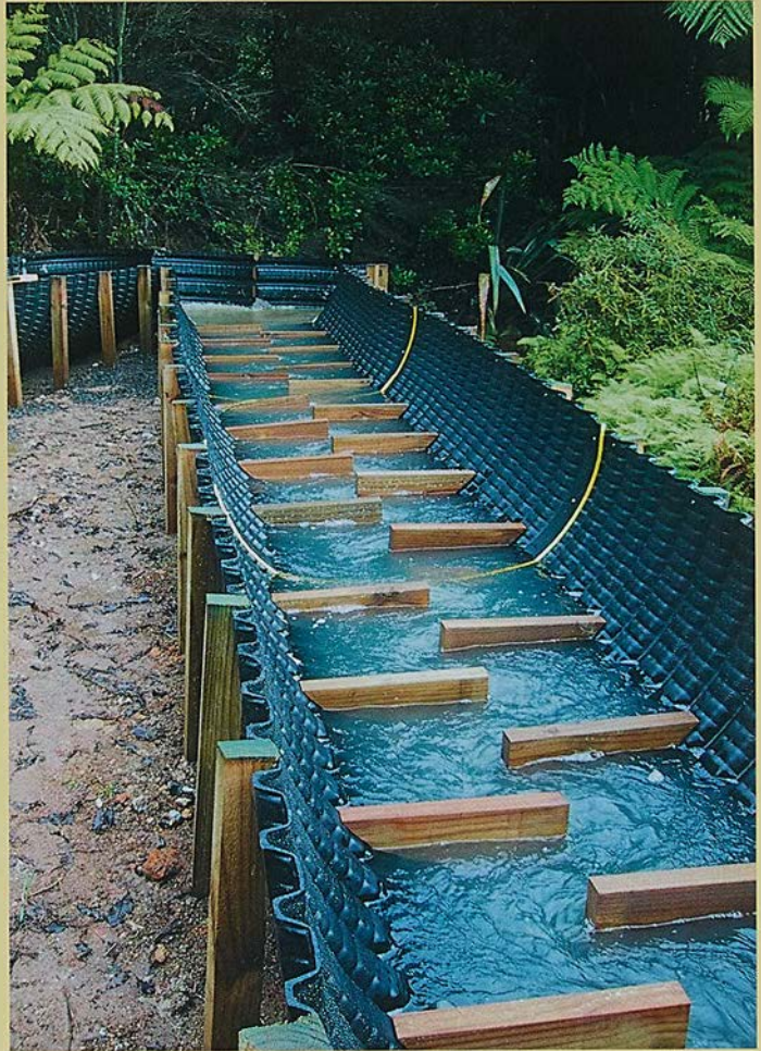
Top opposite page: (Picture 1) A culvert that allows fish to pass under a road.
