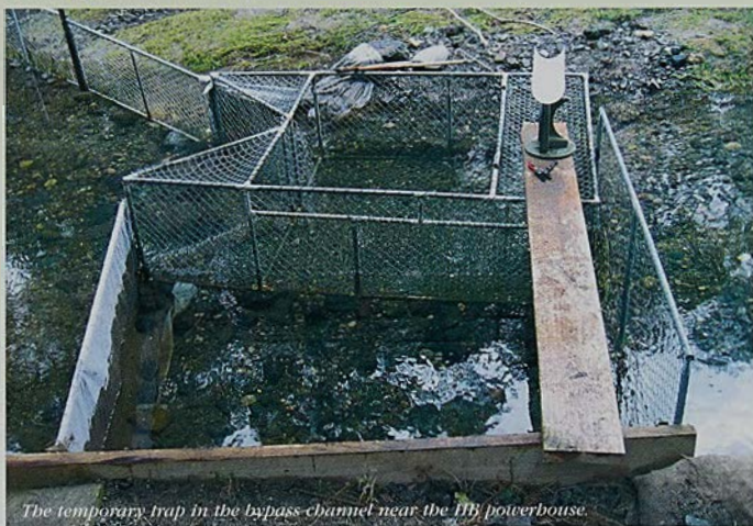
The temporary trap in the bypass channel near the HB powerhouse.
