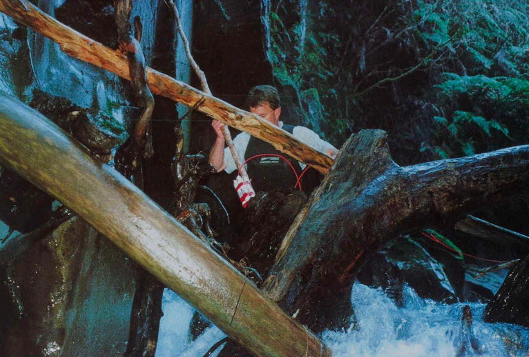
Glenn Maclean prepares to push a charge deep into the log jam
