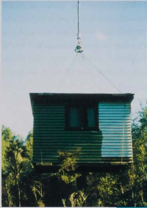
Derek Lowe approaches with the hut, using the tops of the manuka to stop the hut swinging before placing it on the site bearers.
