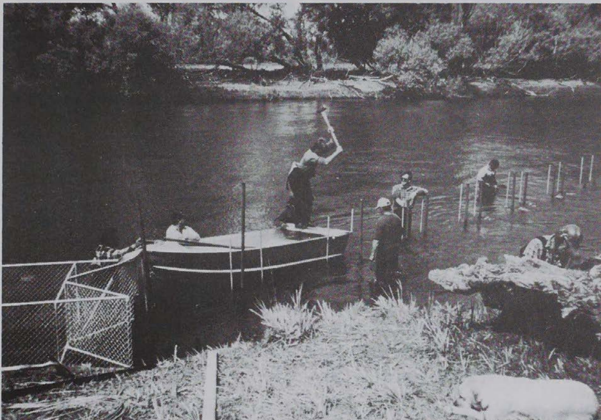
Fisheries staff drive the supports for the screens to sit against. The cage trap sits in the foreground.
