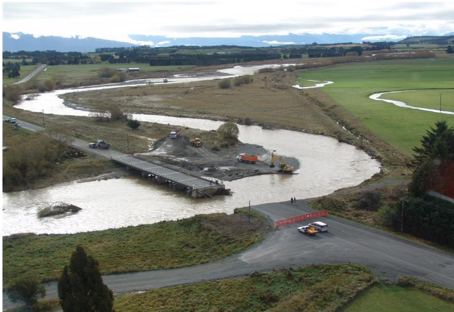
Figure 1: Photo of Whitestone River (SH 94) Bridge Washout taken April 2010.
