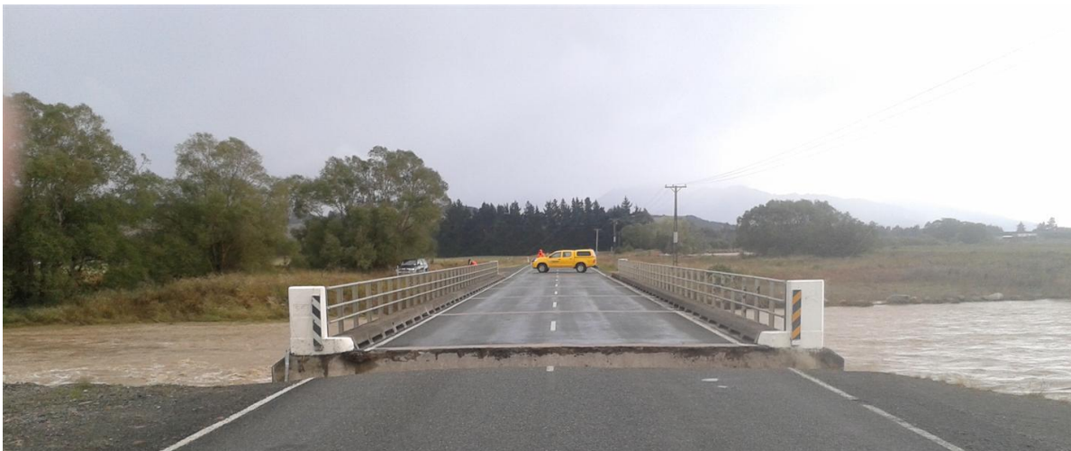
Photo 4: Whitestone River bridge washout 10 January 2013.
