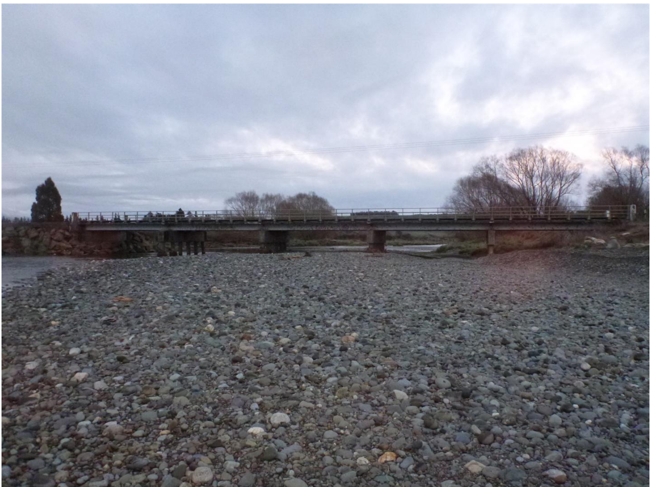
Above: Looking downstream to bridge (2014)
