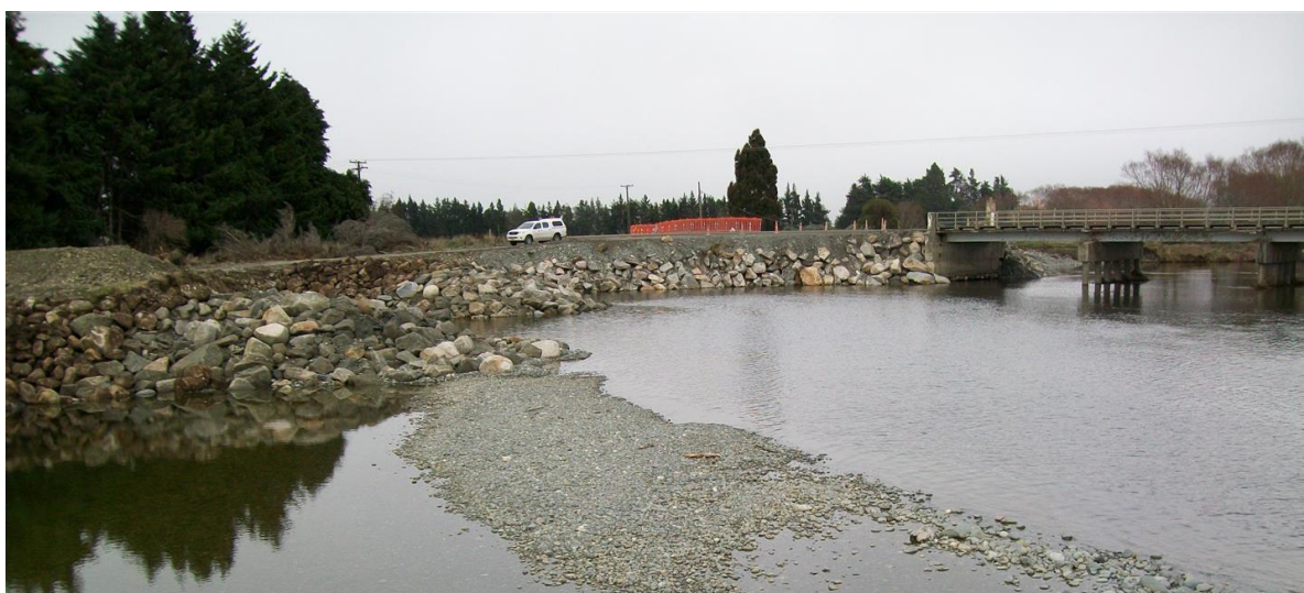
Figure 3: Photo of Erosion Protection Groynes and Bridge Washout Reclamation Constructed 2010.
