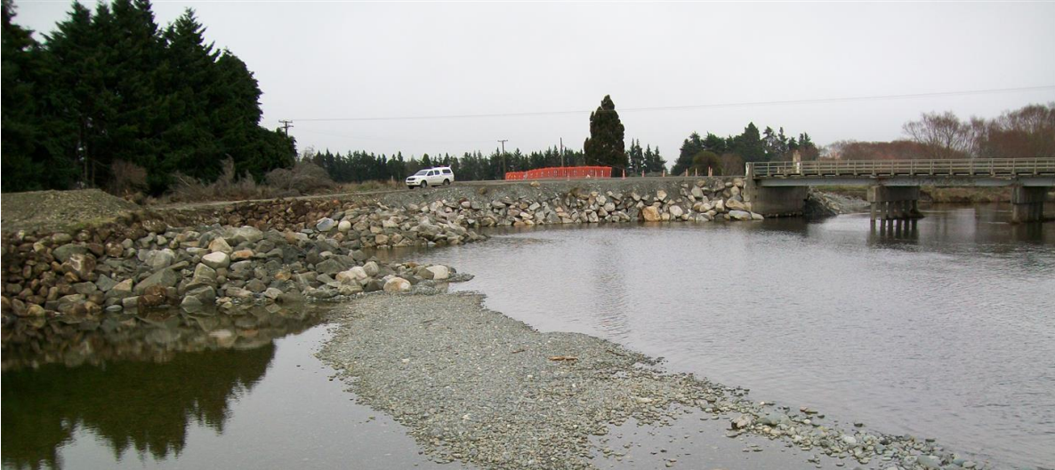
Photo 2: Erosion protection groynes and bridge washout reclamation constructed in 2010.
