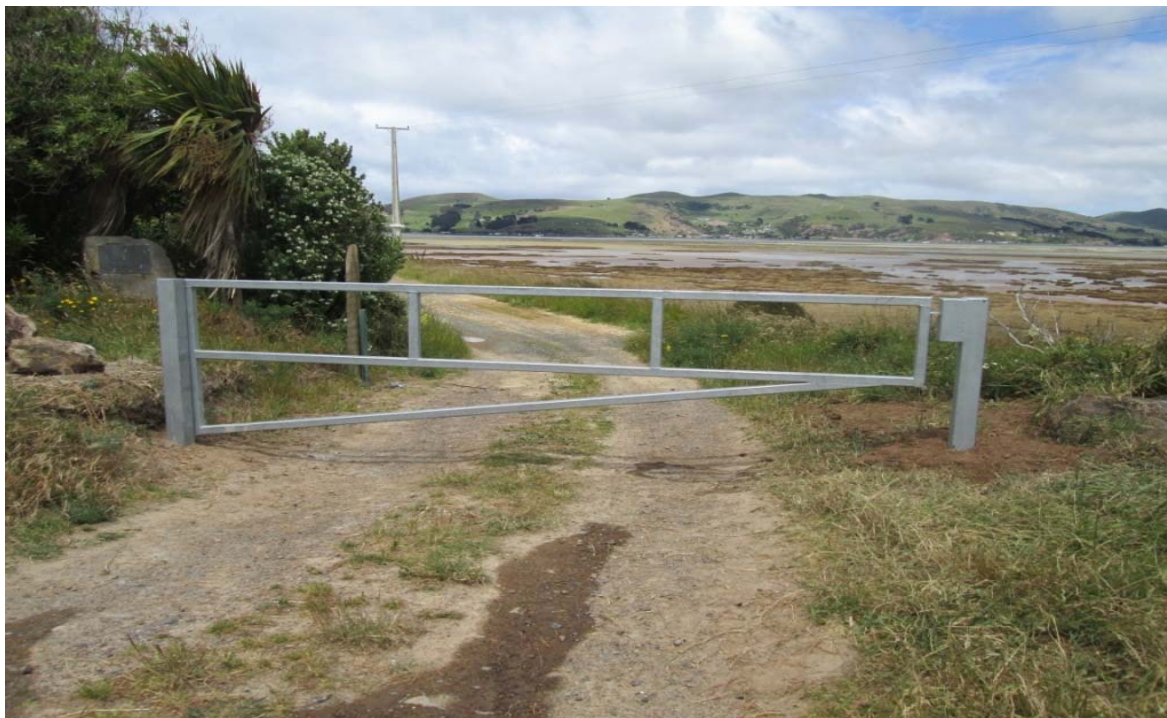
Figure 2: Photo of gate (December 2015) as shown on Appendix G map
