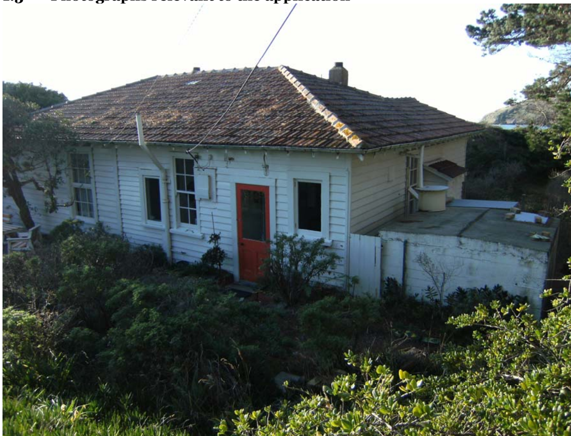
Figure 1: Cottage/pilot house No.3 (July 2015)
