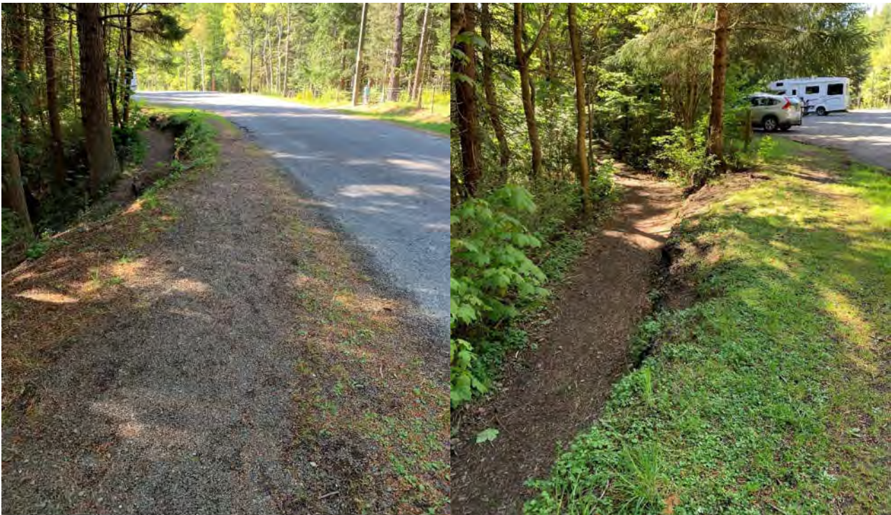
Photograph 11: Alternate Pedestrian Paths Along Jollies Pass Road (Left: Route Along the Edge of the Road; Right: Route Along the Ledge/Internal Part of the Forest)
