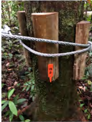
Tree 18A and 18B are bracing Tree 18
