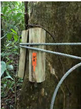
Tree 25A and 25B are brac ng Tree 25
