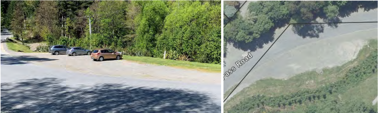
Photograph 7: Area 7 Parking (Left: View from the Northwest; Right: Aerial)
