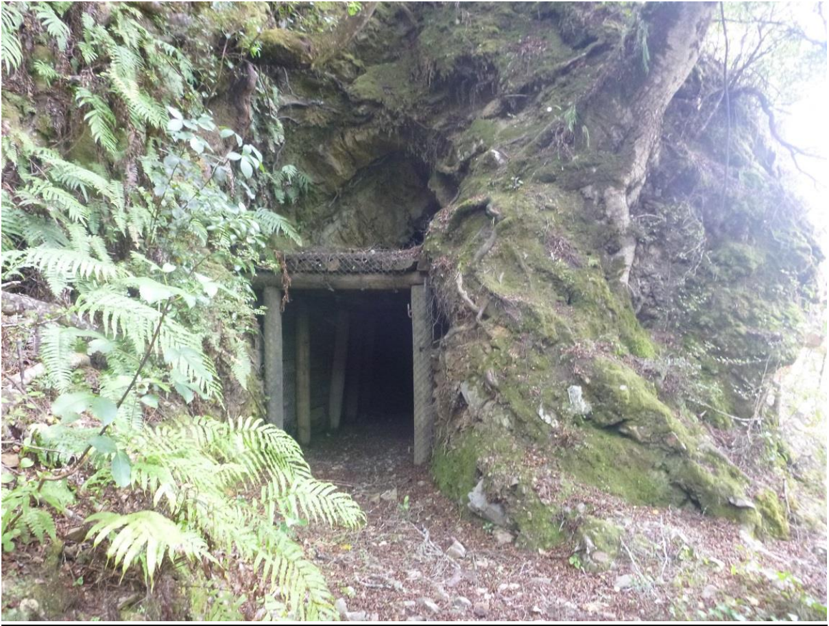
Photo 1: Eastern tunnel portal, dimensions of approximately 2.3 metres wide by 2.2 metres high.
