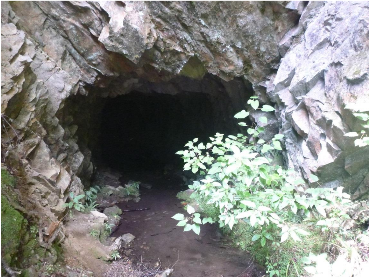
Photo 2: Western tunnel portal, dimensions of approximately 2.7 metres wide by 2.2 metres high.
