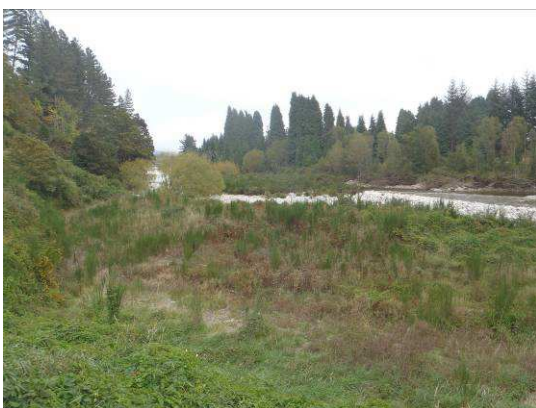
View of power station outlet.
