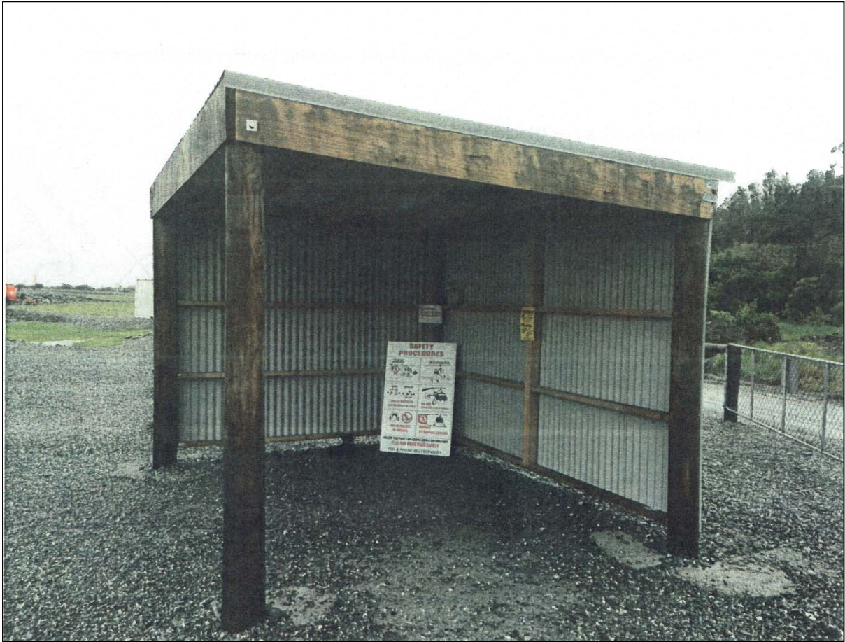
Figure 20 - Example of what the Shelters (two are proposed) for waiting passengers would look like. Note this is indicative only.
