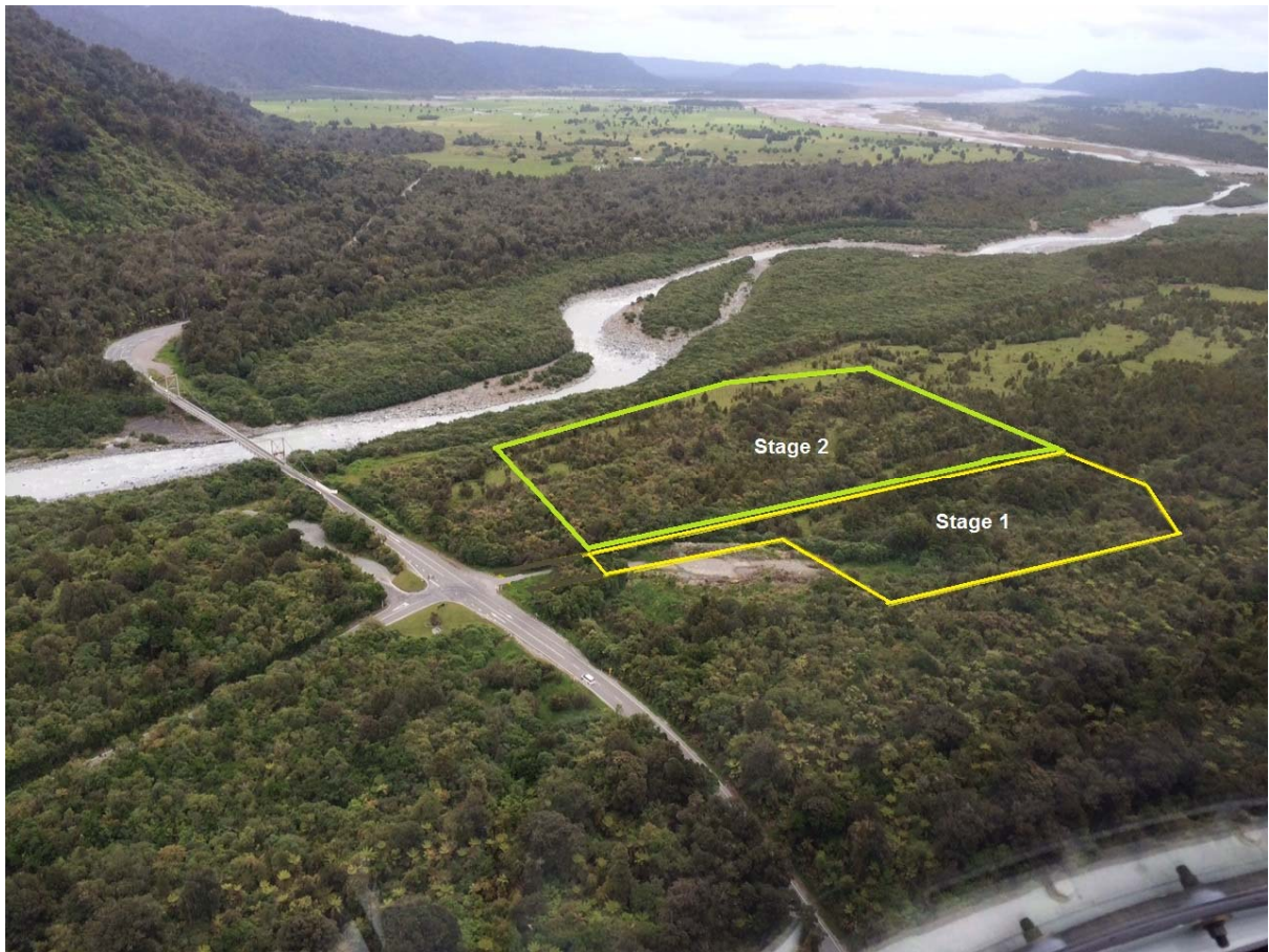
Figure 13 - Aerial view of the site from a helicopter. The yellow lines are the approximate boundaries of the site Stage 1 and the green outline Stage 2. The photo is taken east of the site (approximately over SH6, the Road is visible) looking southwest.
