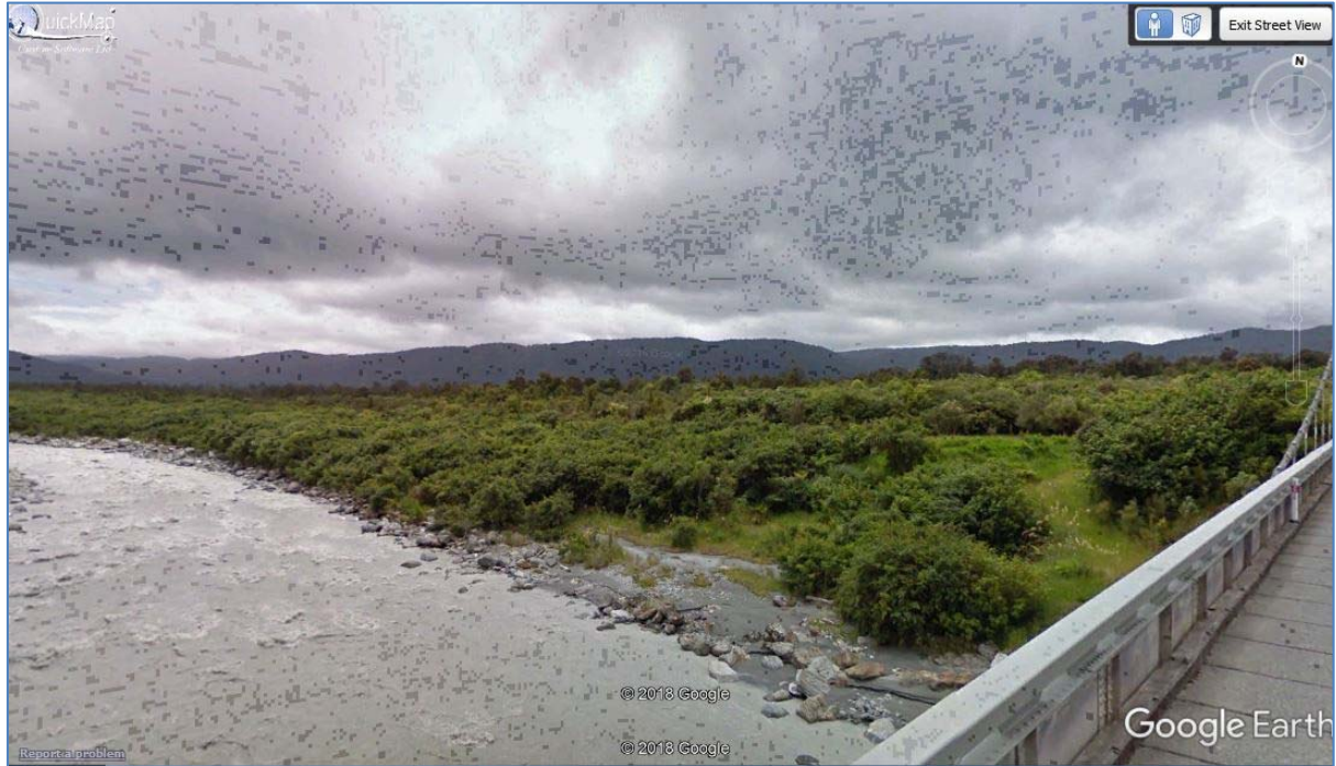
Figure 17 - photo from further along the SH6 Bridge looking north over the site. (Source: Google Earth)
