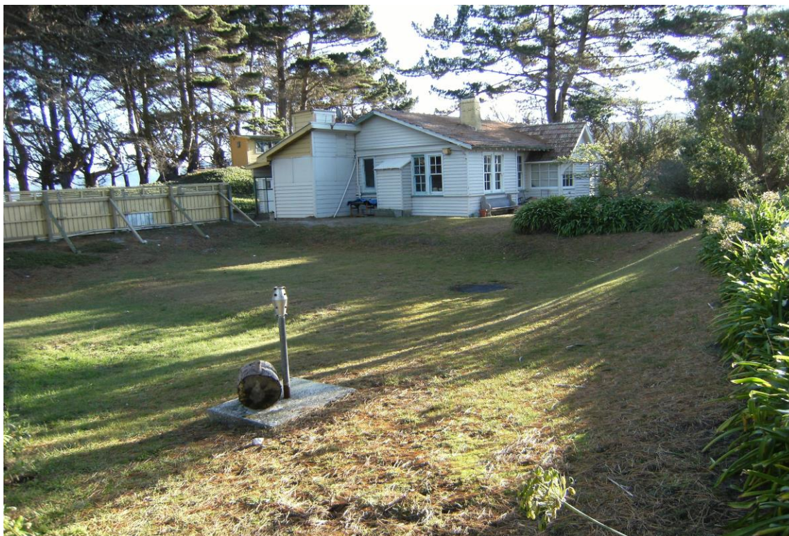
Figure 1a: Cottage/pilot house No.2 photo (July 2015)
