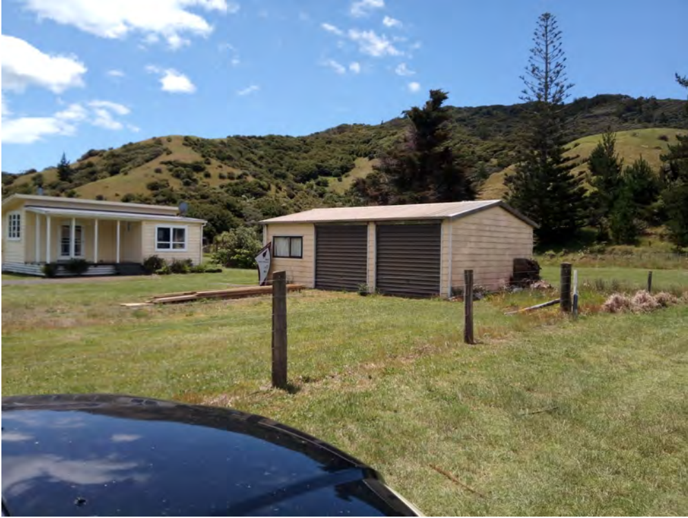
Cottage and workshop
