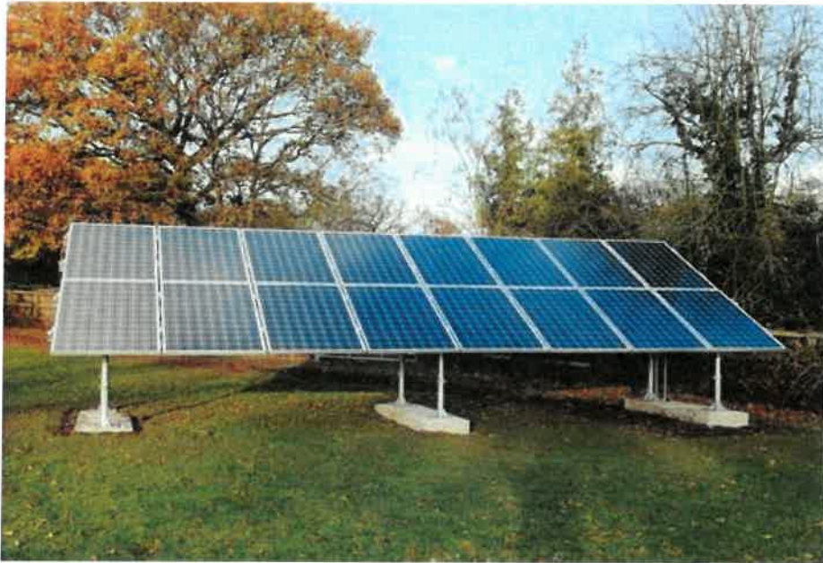
Figure 6: Example of 16 panel, ground mounted system
