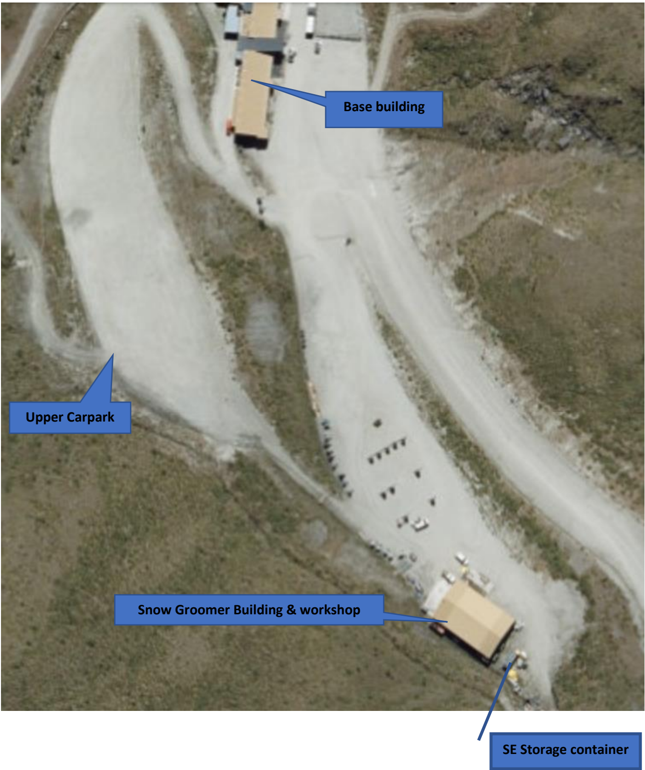
Figure 14 Aerial View of Base Building relative to Snow Groomer & workshop building
