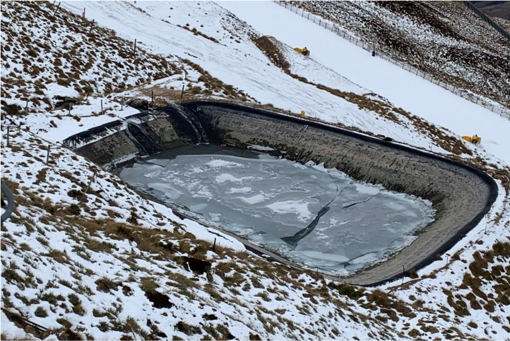
Figure 36 Snow making reservoir (main)
