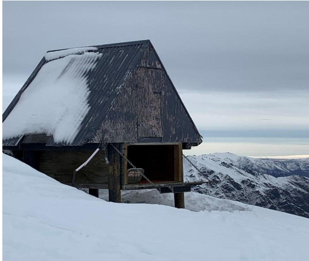
Figure 64 Small 'A' frame Patrol Equipment shed
