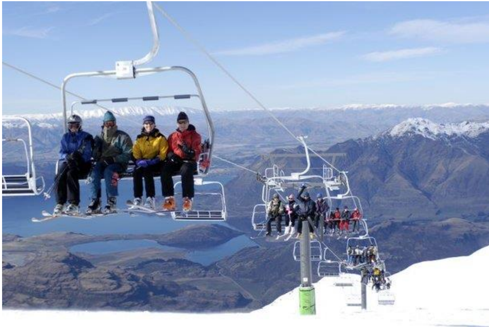
Figure 61 Quad Chair Lift – including pylons
