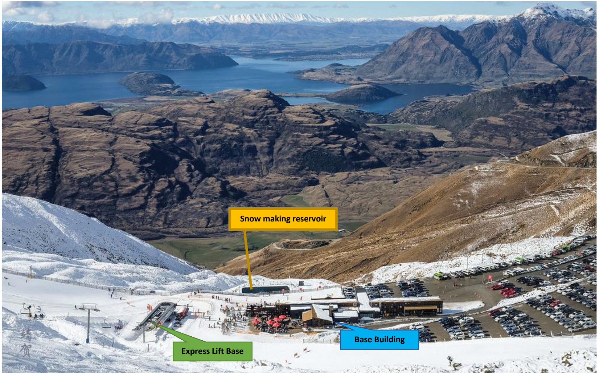
Figure 18 Overview of Treble Cone Home Basin infrastructure
