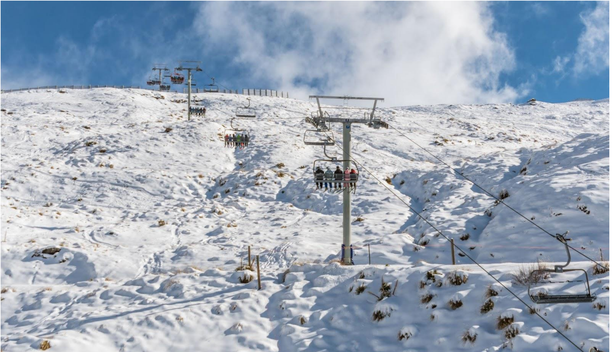
Figure 43 Express Lift – pylons
