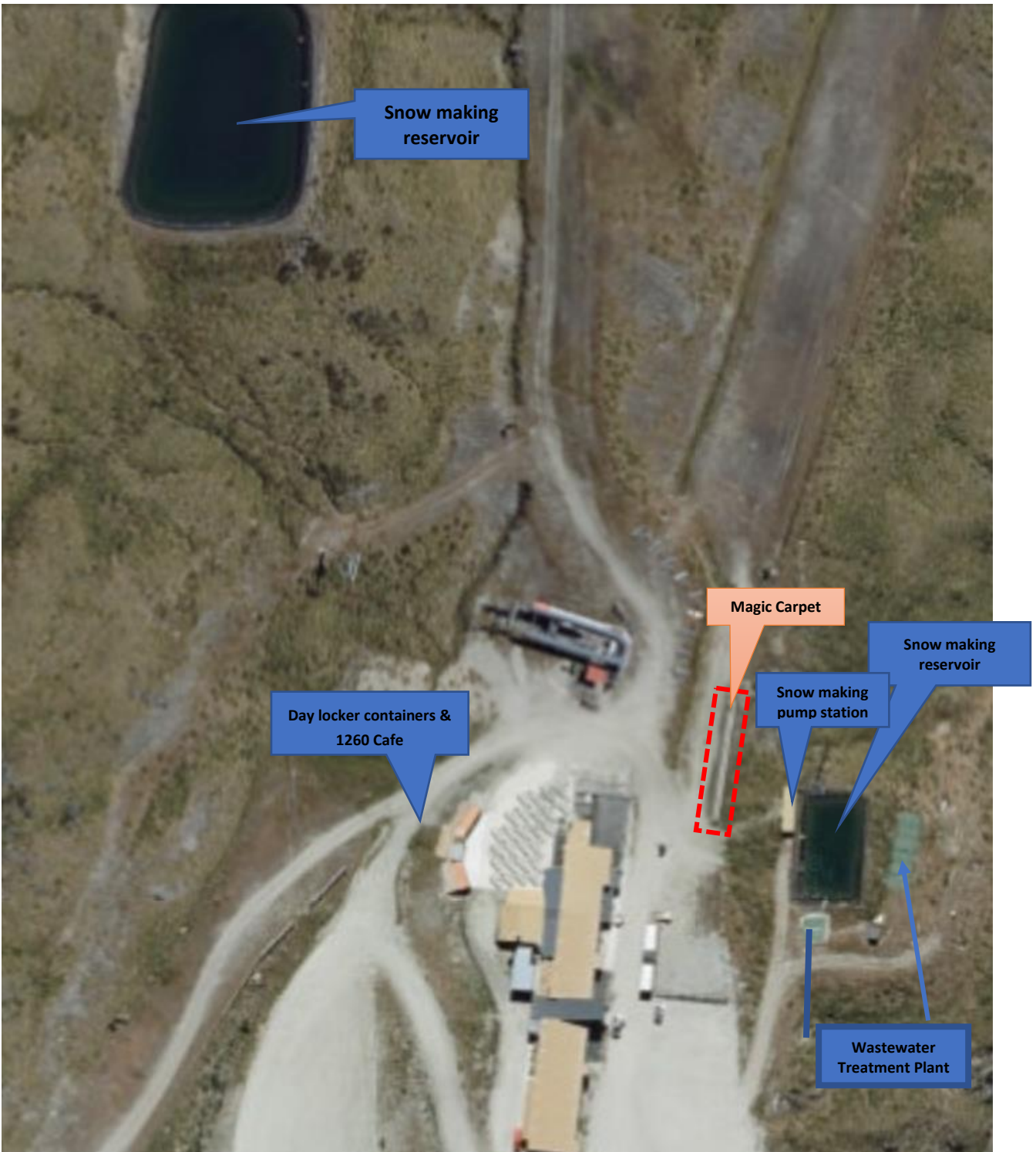
Figure 13 Aerial View of Base Building and surrounding infrastructure
