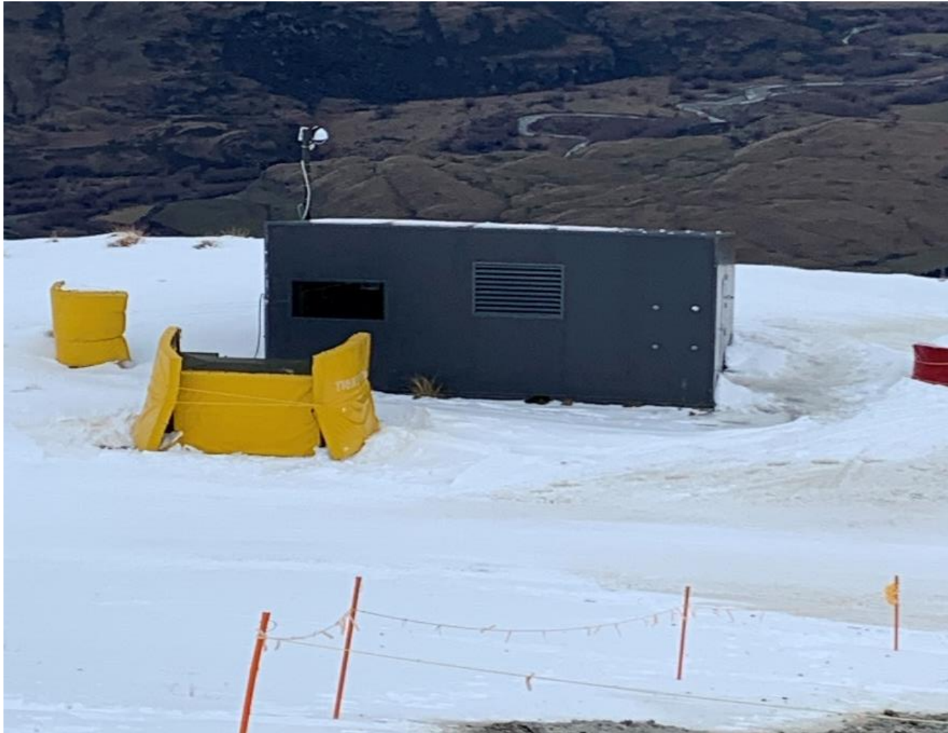
Figure 57 Mid Mountain Booster pump station
