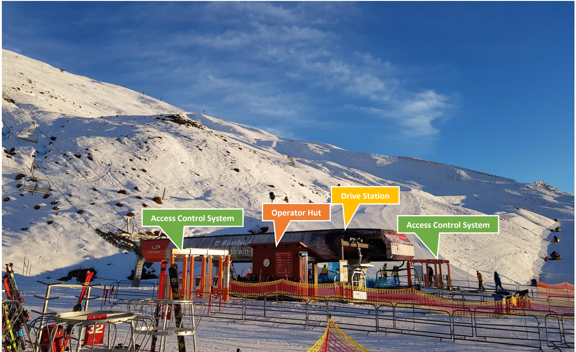
Figure 42 Express Lift – base incl operator shed plus 2x access control systems
