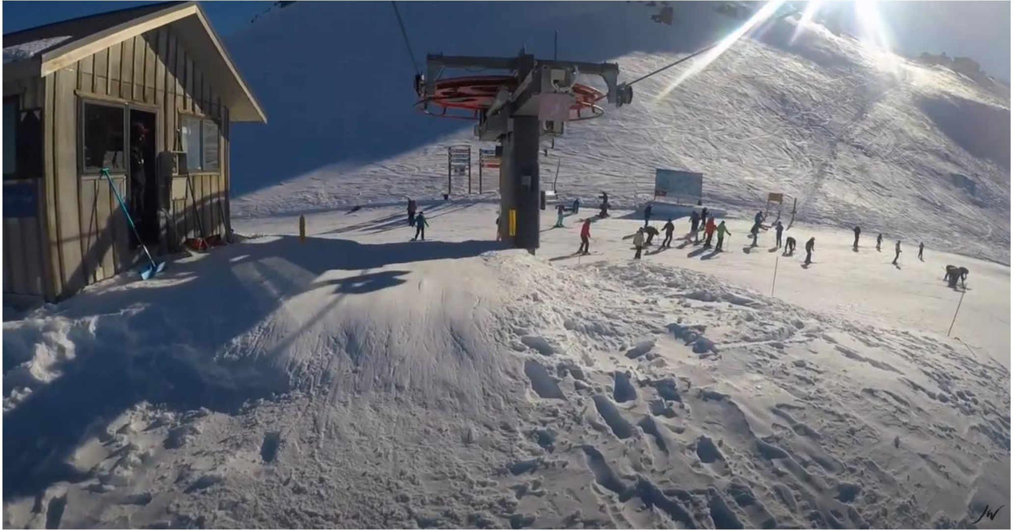
Figure 63 Top of Quad lift – return station and operator / patrol hut
