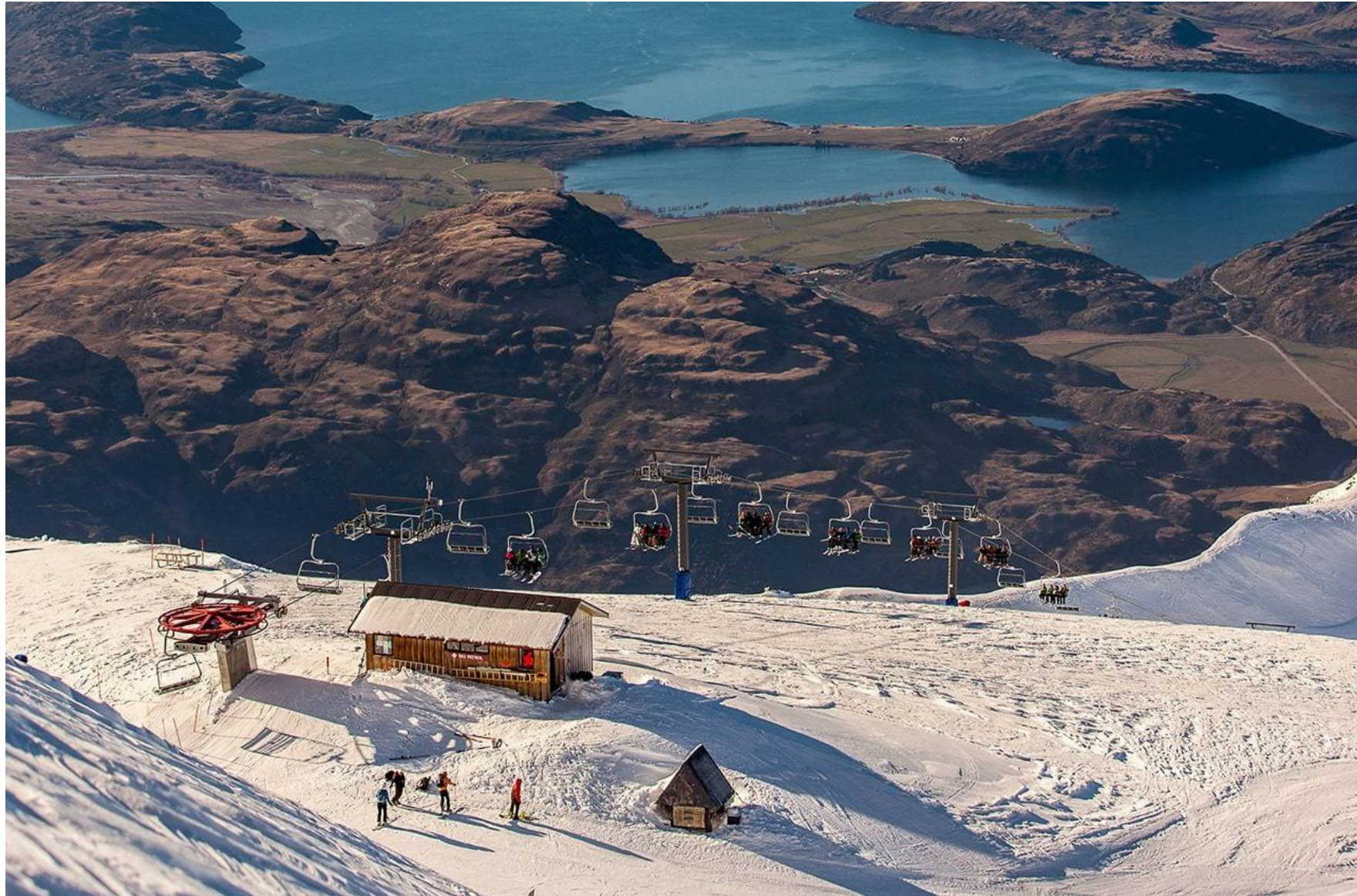
Figure 62 Top of Quad lift – return station; operator / patrol hut and small 'A' Frame Patrol Equipment Shed
