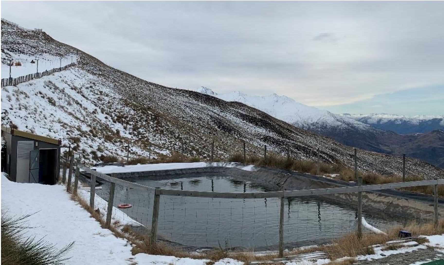
Figure 34 Snow Making Reservoir (bottom) and Pump House (Main)
