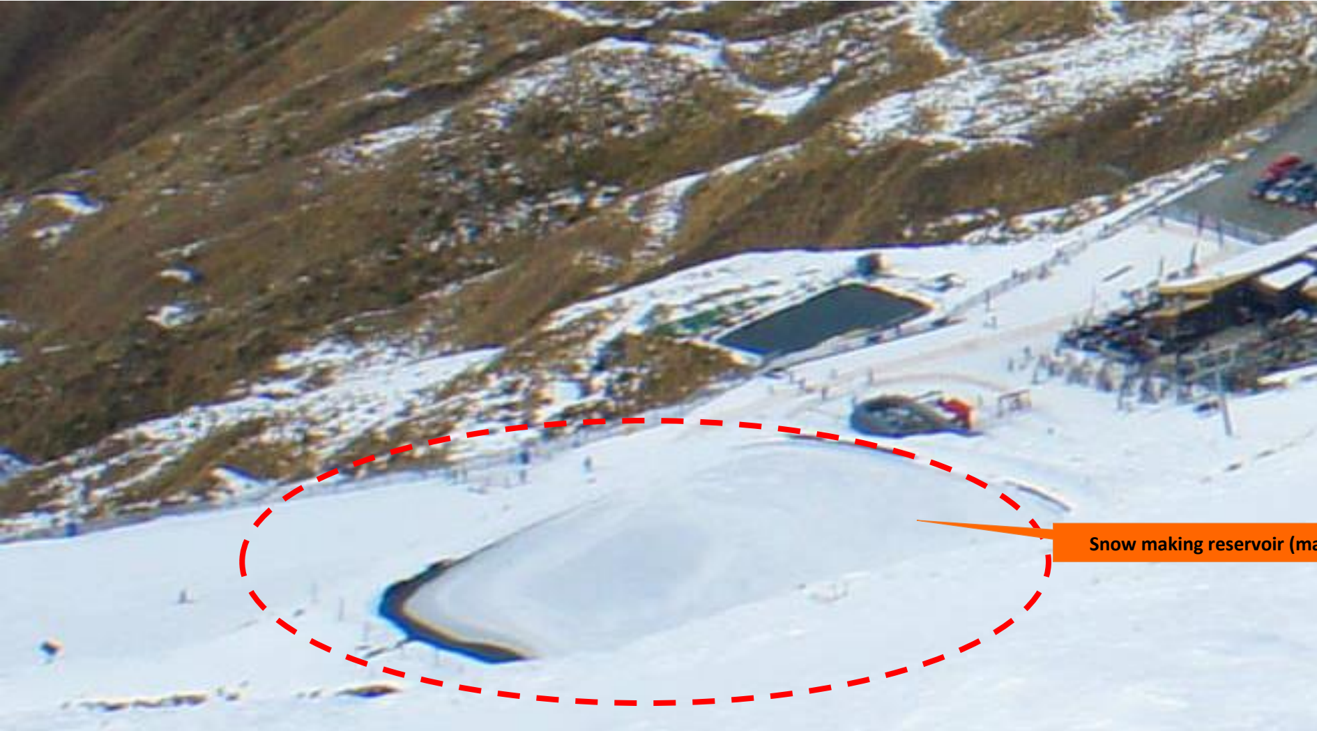
Figure 35 Snow making reservoir (main)
