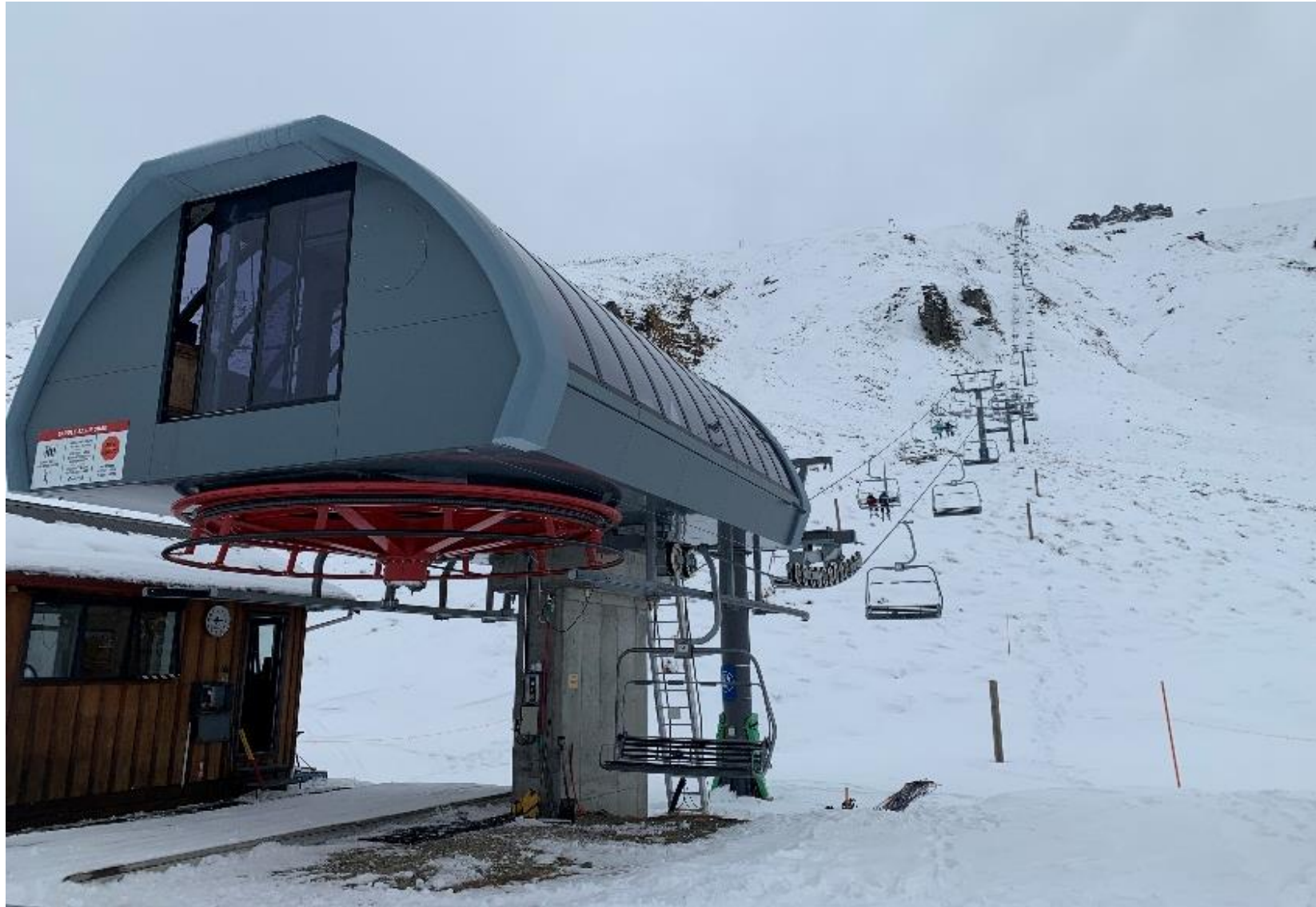
Figure 60 Lift Machinery Shed at Quad Base (drive)
