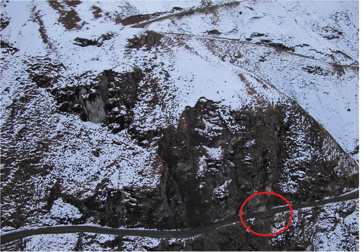
Figure 5 & 6 Access Road Bridge
