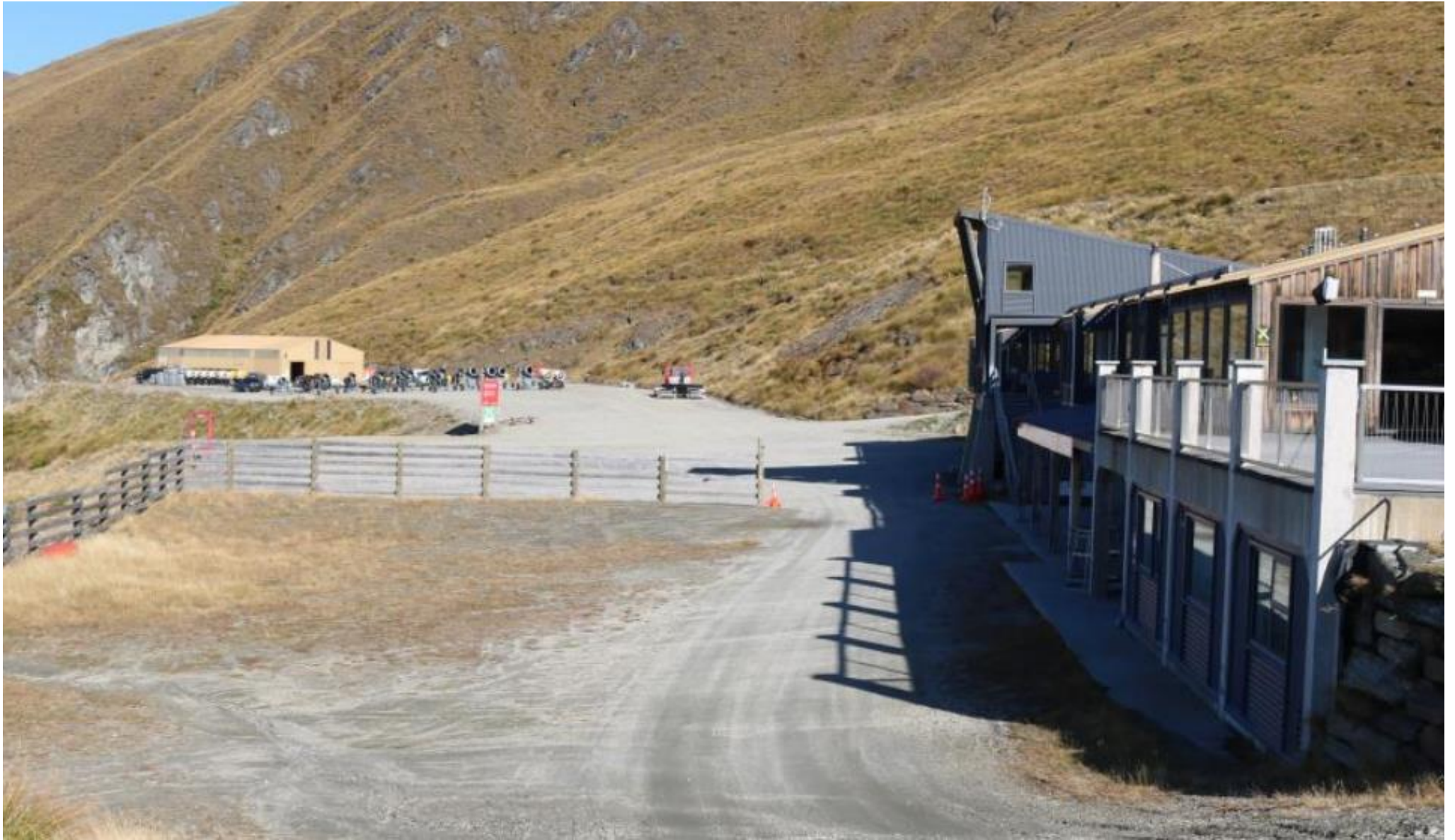
Figure 19 Snow Groomer / Workshop Building relative to Base Building
