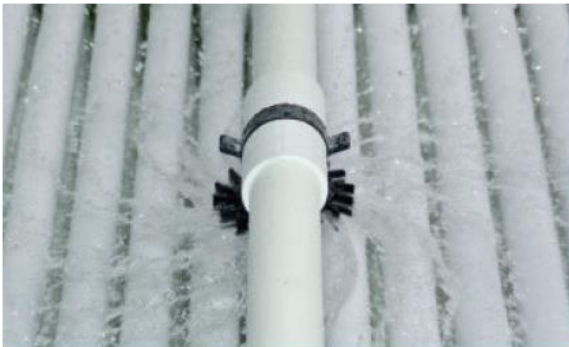
Figure 6. Spray nozzle inside AX100 Pod
