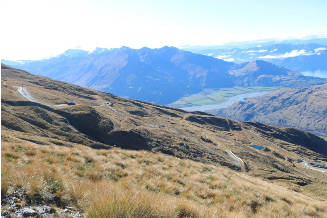
View of Home Basin including chairlift, lunch hut, reservoir, piste runs, vehicle access and top car park and base building bottom right.
