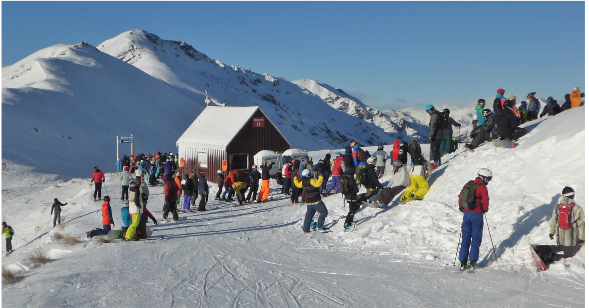
Figure 53 Old lift tow shed (Saddle) – (converted to a toilet block)
