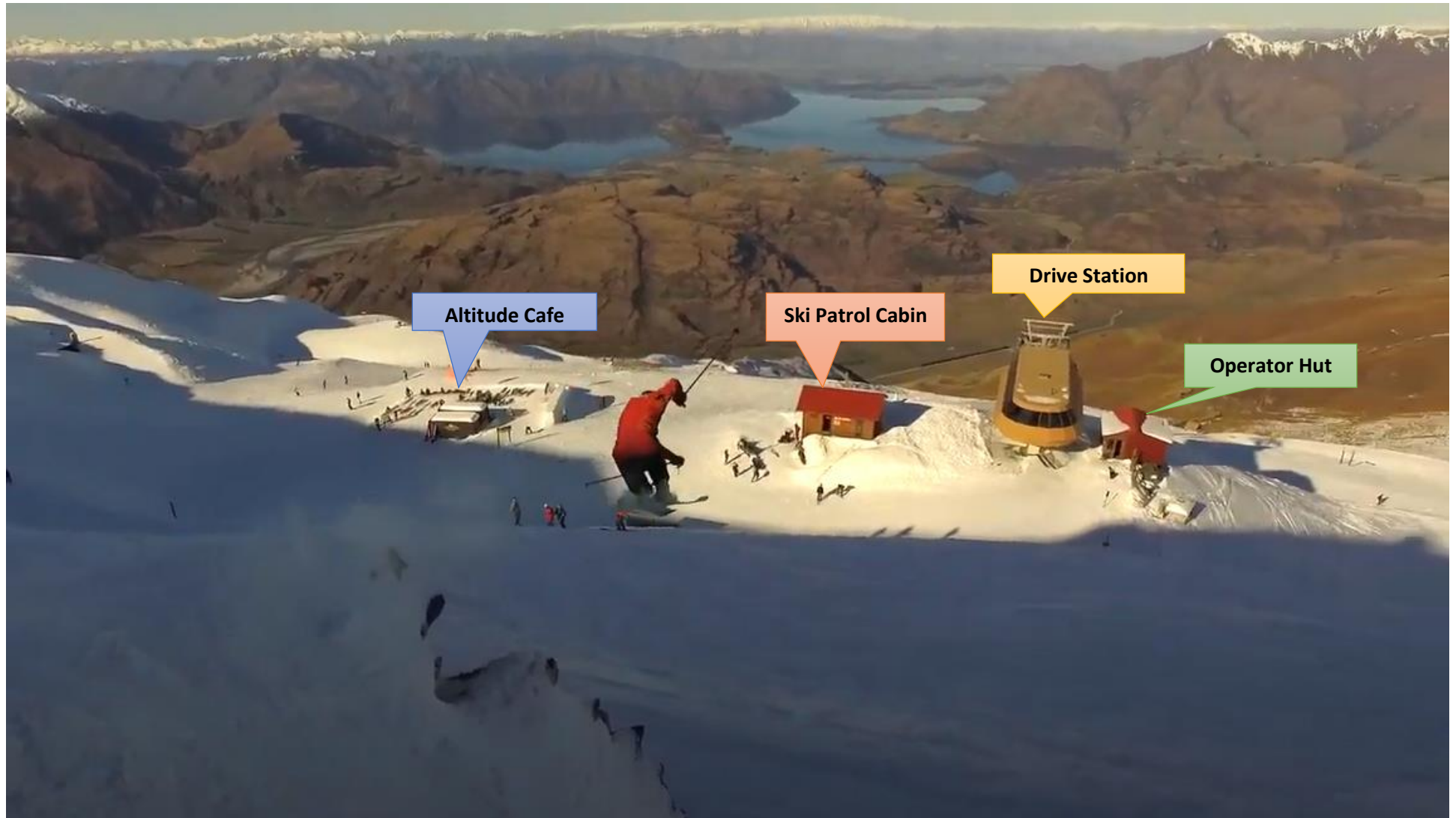
Figure 45 Top of six-seater express lift – Drive Station + Ski Patrol Cabin + Altitude Cafe
