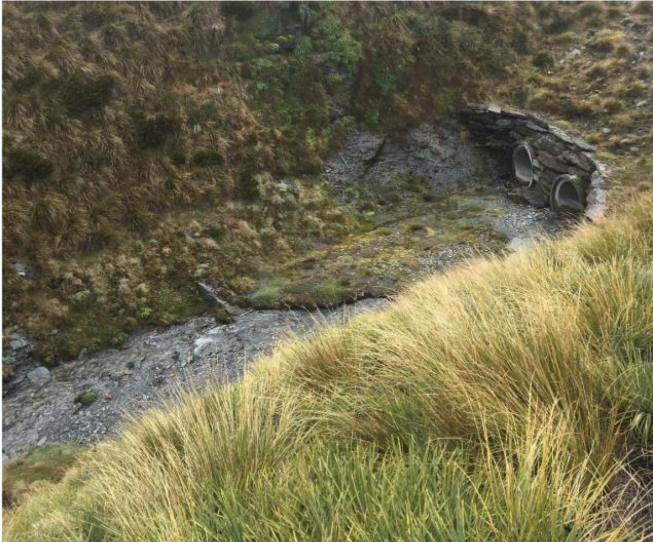
Figure 10 – Example of Culvert
