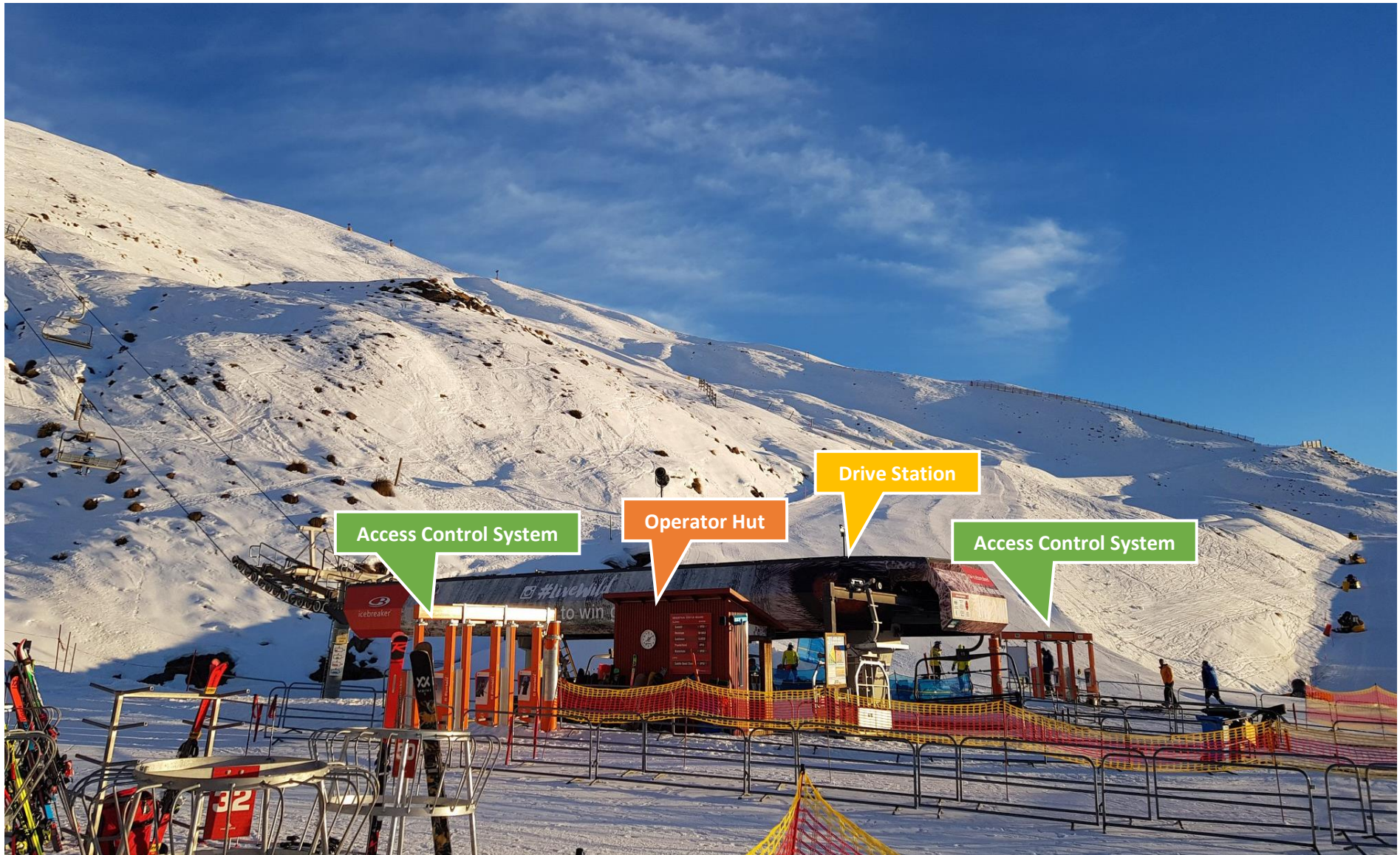
Figure 43 Express Lift – base incl operator shed plus 2x access control systems
