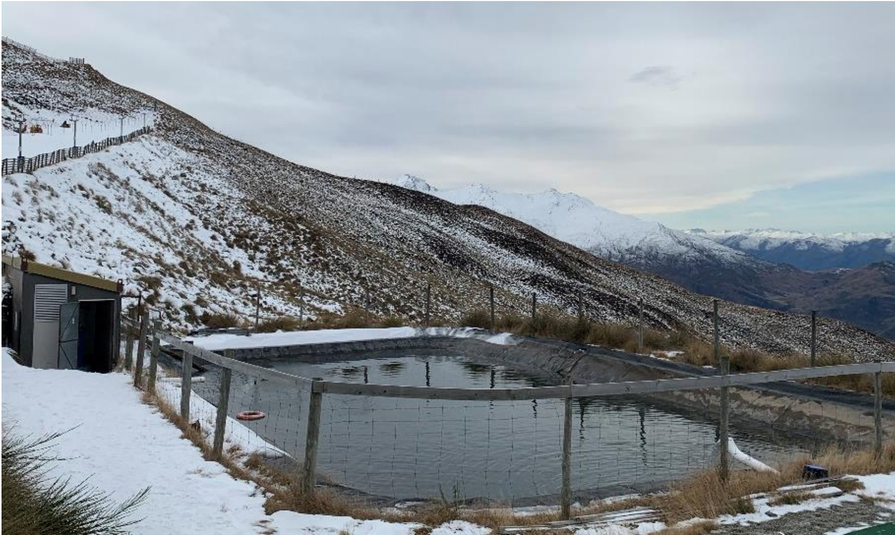
Figure 37 Snow making Reservoir (bottom) incl Main Pump House
