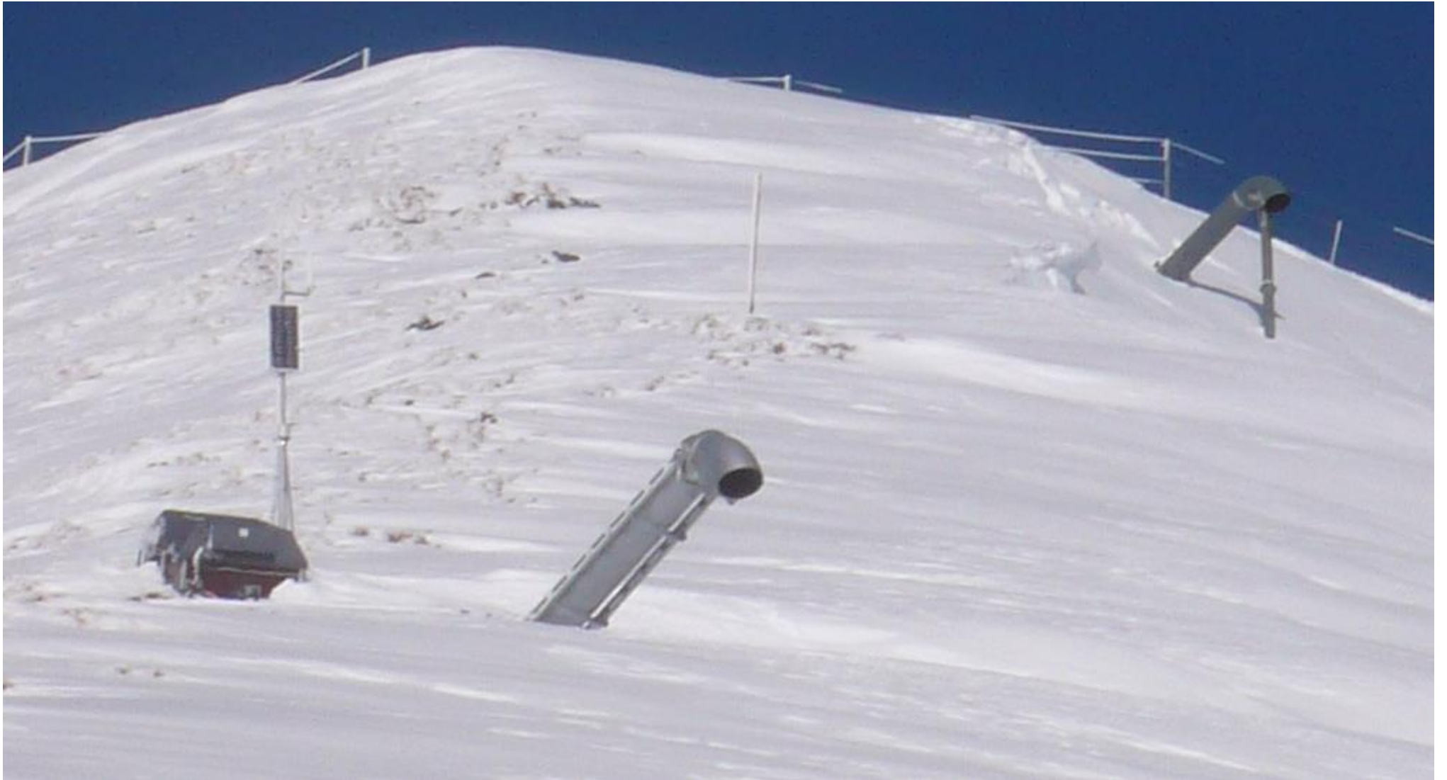
Figure 67 Proposed Avalanche Protection Devices (Gazex)
