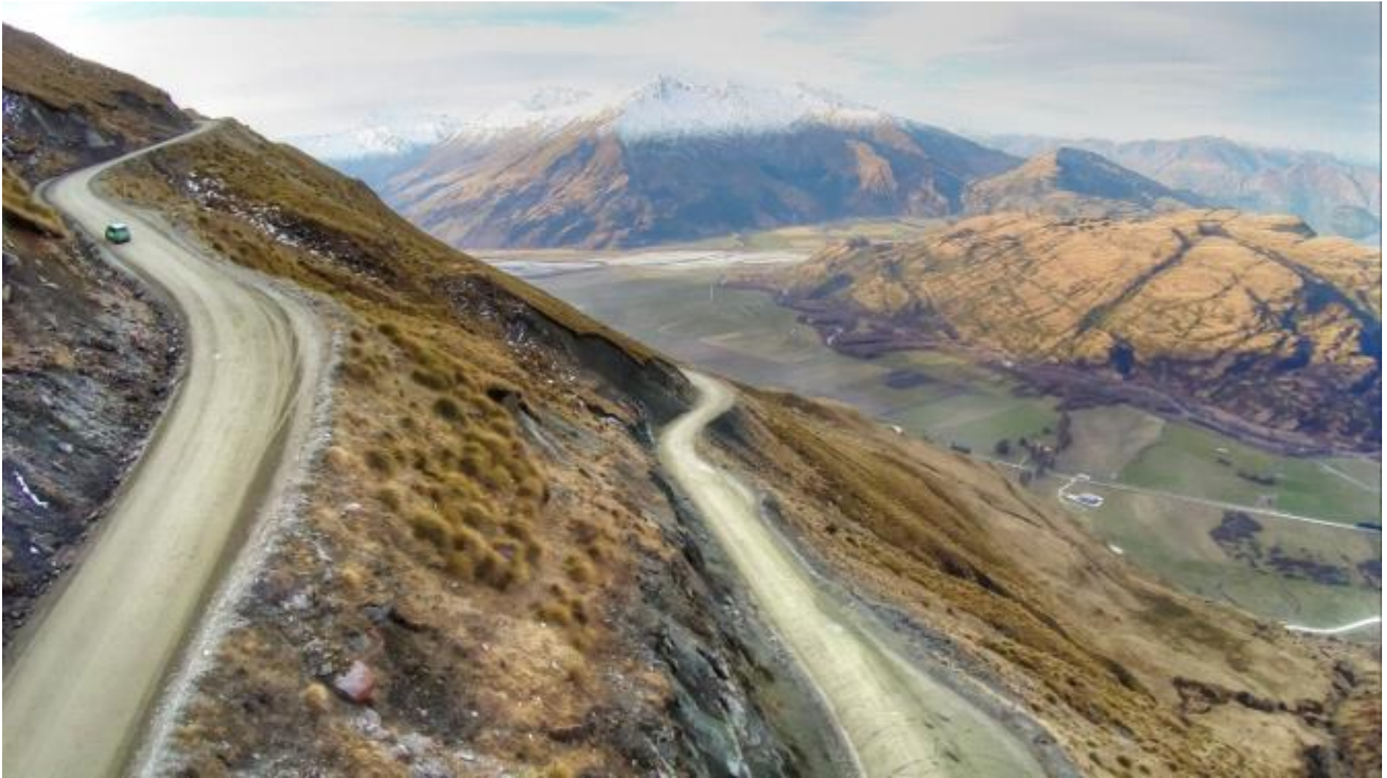
Figure 6 Treble Cone Access Road
