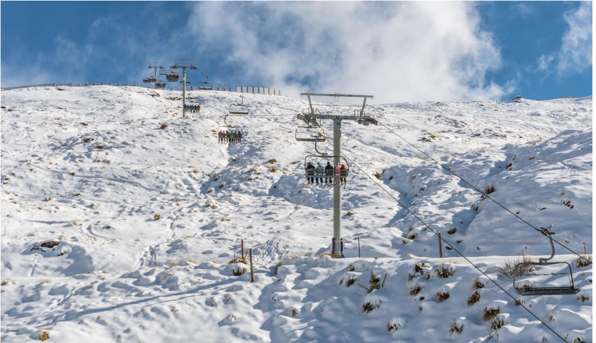
Figure 44 Express Lift – pylons
