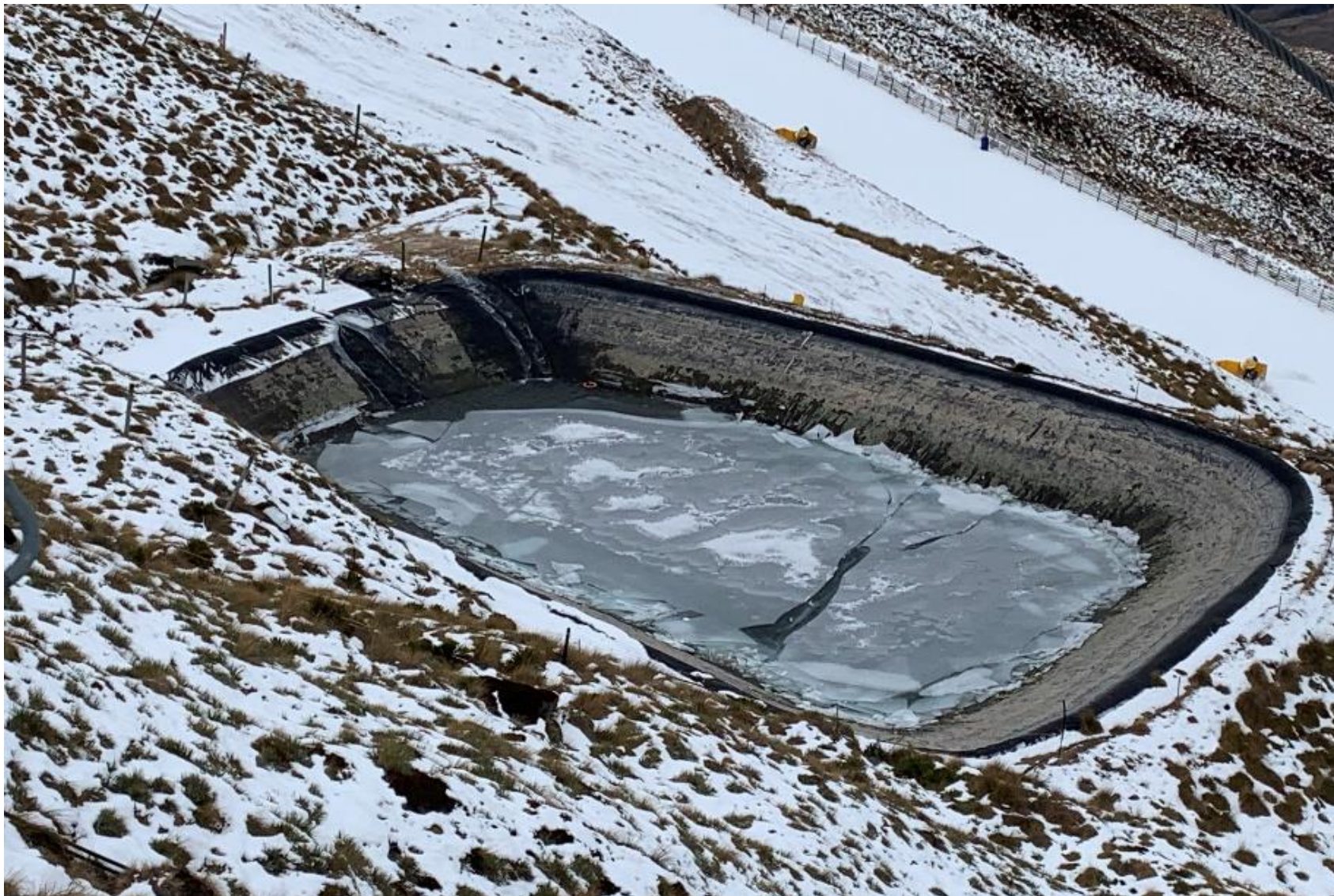
Figure 39 Snow making reservoir (main)
