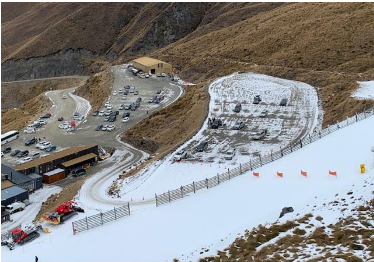
Figure 17 Base car parks & top of Access road.
