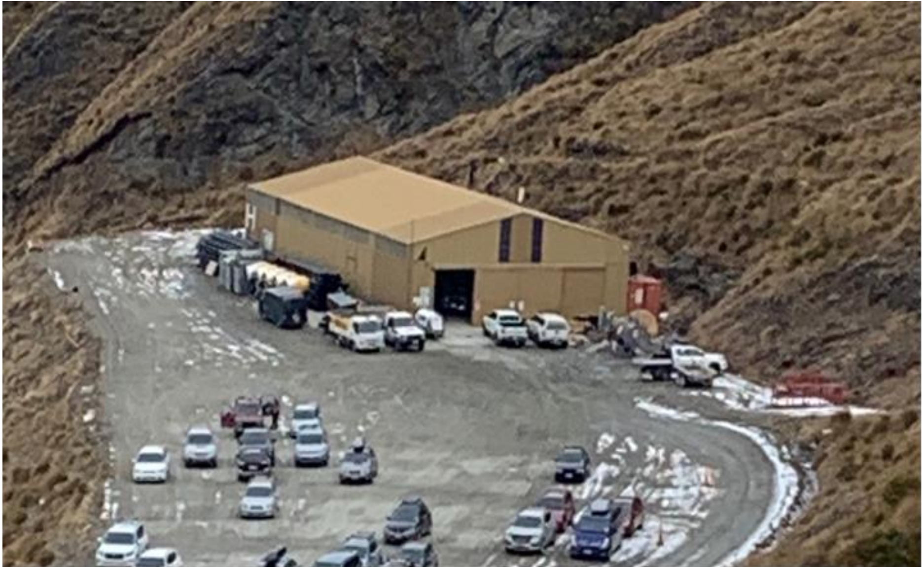
Figure 20 Snow Groomer Building incl workshop
