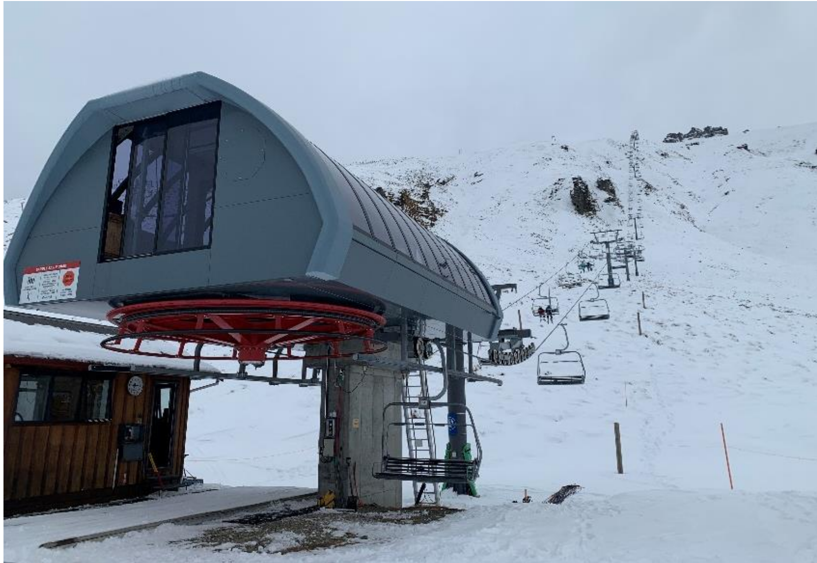
Figure 58 Lift Machinery Shed at Quad Base (drive)
