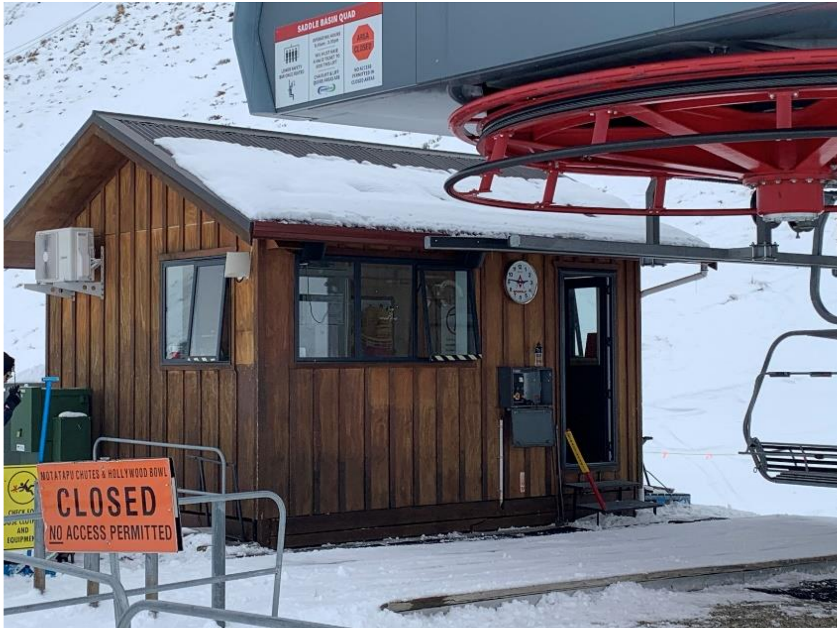
Figure 57 Base Quad lift operator hut
