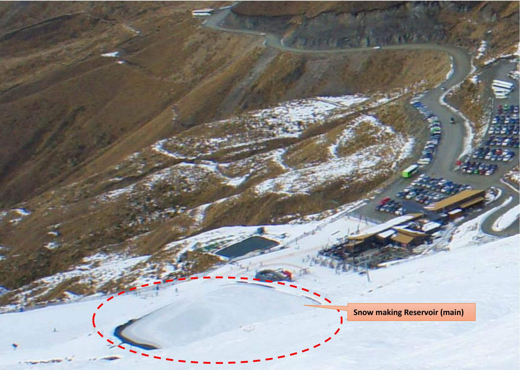
Figure 38 Snow making Reservoir (main)
