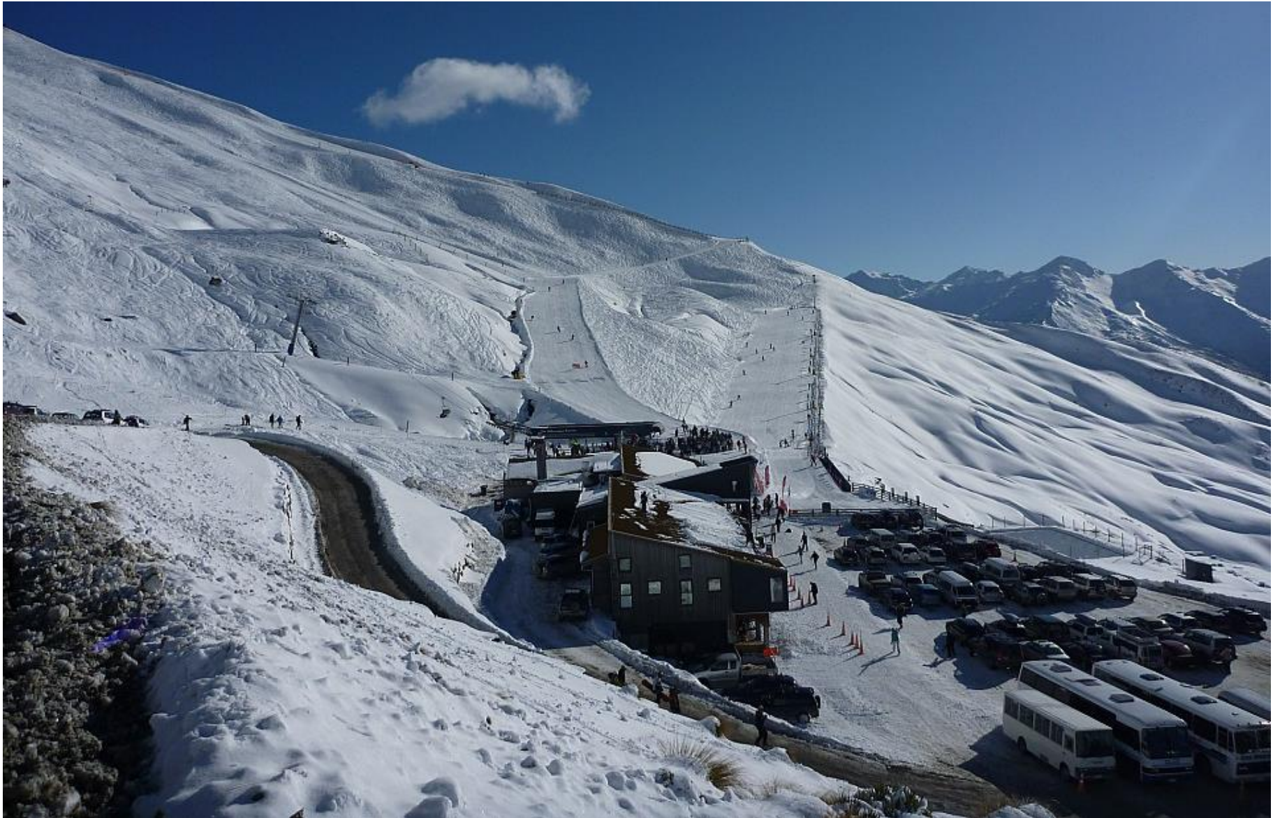
Figure 15 Top end (Northern End) of carpark with road up to Upper Car park on left
