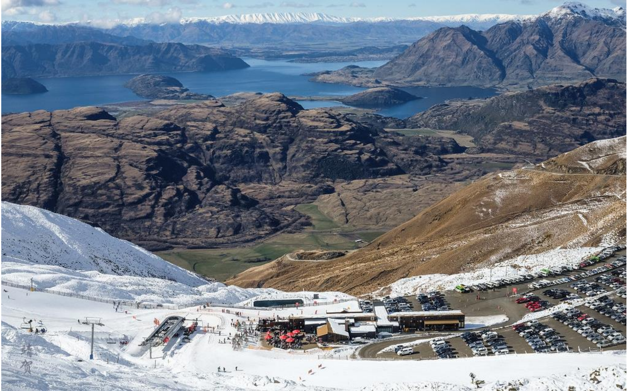
Figure 19 Overview of Treble Cone Home Basin infrastructure
