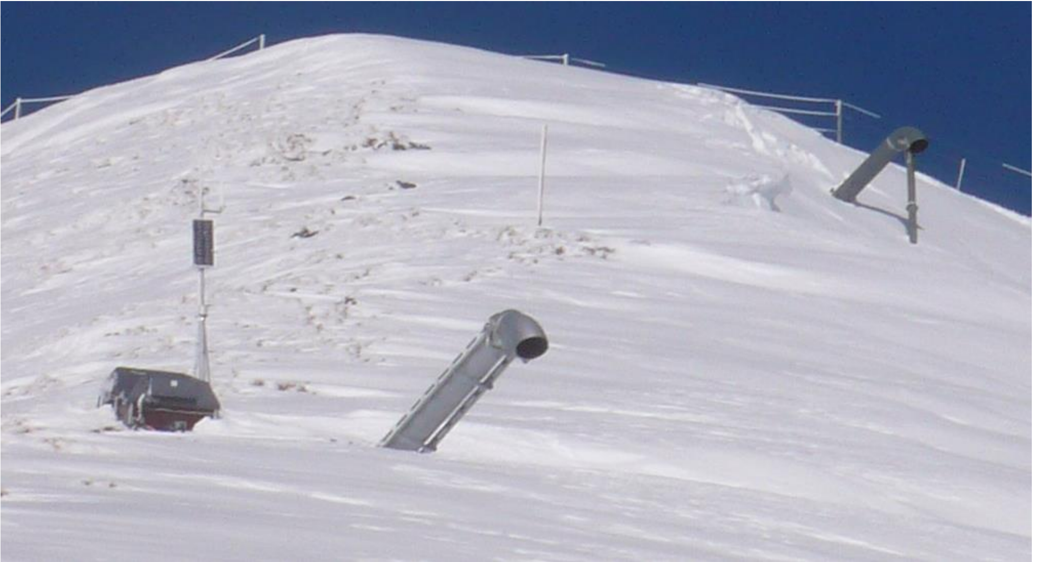
Figure 41 Proposed Avalanche Protection Devices (Gazex)
