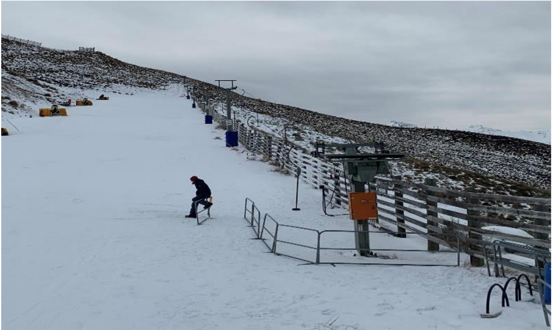
Figure 25 Base of Platter Lift
