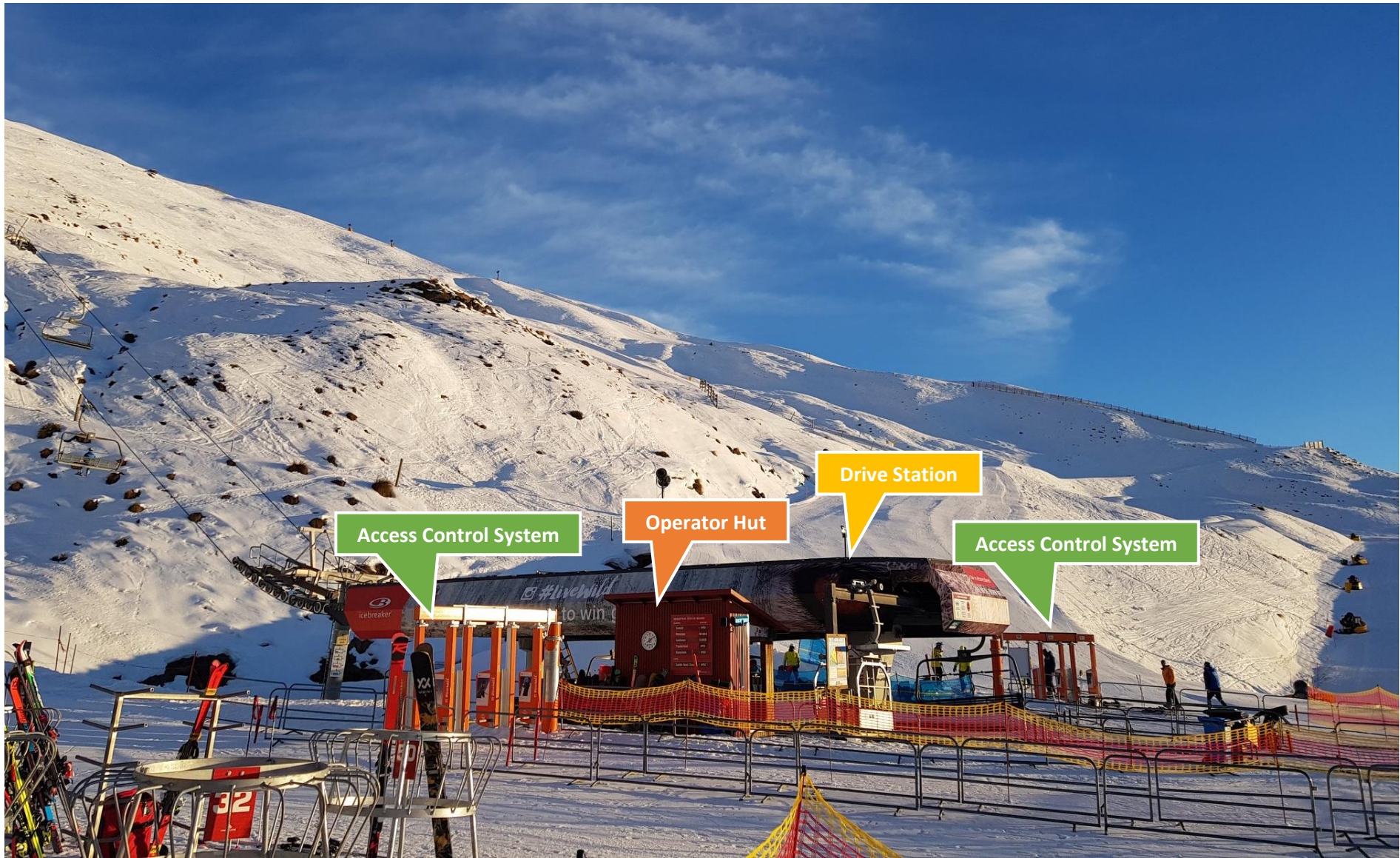
Figure 27 Express Lift – base incl operator shed plus 2x access control systems
