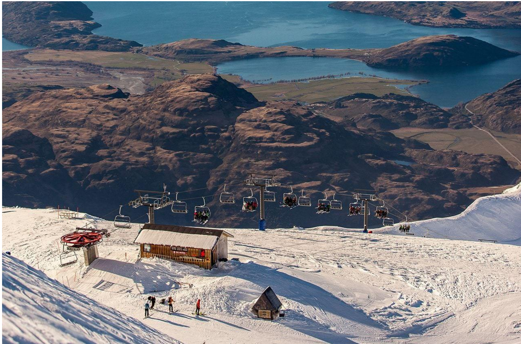
Figure 36 Top of Quad lift – Return station, operator / patrol hut and small 'A' Frame Patrol Equipment Shed
