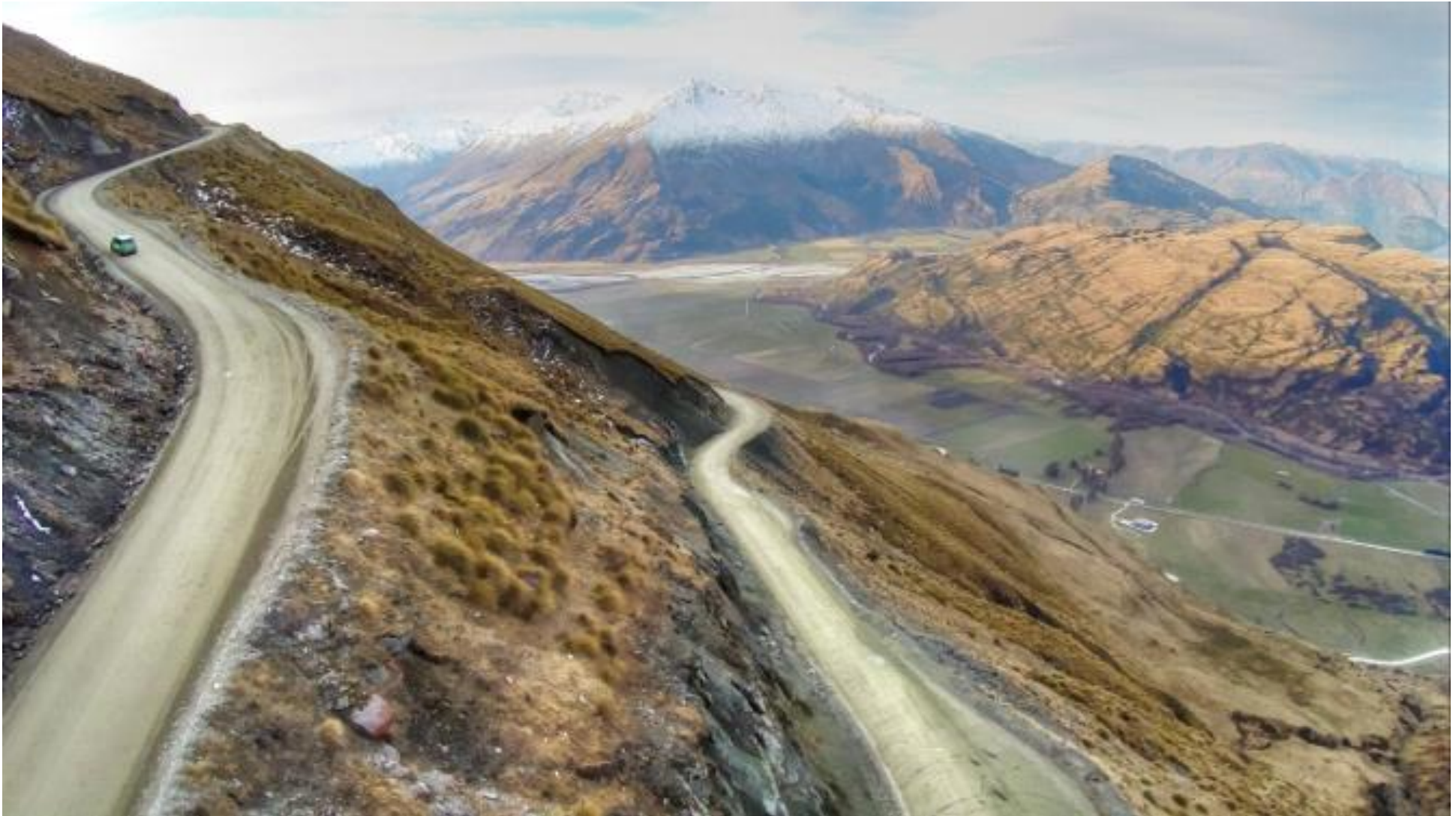
Figure 6 Treble Cone Access Road within Motatapu Conservation Area
