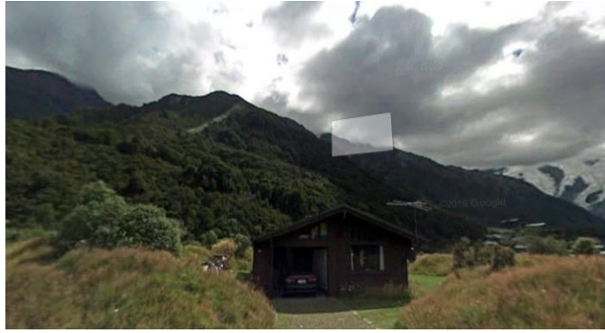
Figure 5 Site 13, 2 Mueller Place
