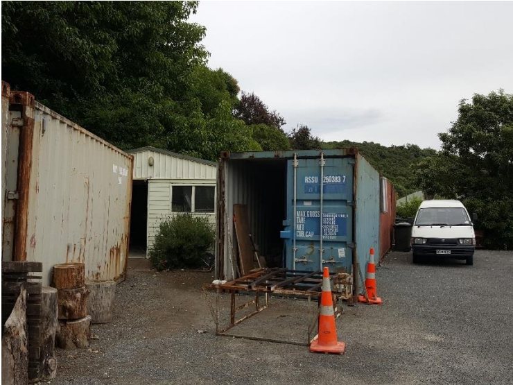
FIGURE 4: EXISTING GARAGE AND CONTAINER PROTECTION
