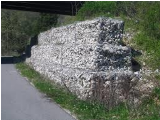
FIGURE 7: INDICATIVE PHOTO OF GABION STRUCTURE NOTE: PROPOSED STRUCTURE IS TWO ROWS IN HEIGHT
