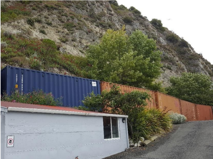
FIGURE 3: EXISTING CONTAINER PROTECTION
