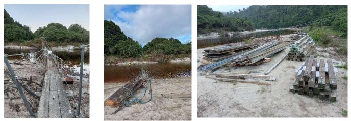
This was a big job. The bridge had over 2000 fixtures, main cables which were 148m long and weighed 360kg each plus a whole lot of wood. The combined weight of material is approximately 12 tonnes (excluding the towers and bridge anchors). All of this was entangled with debris in the river after the storm. Wherever possible, materials will be reused in the new bridge, but regardless, every little piece must be taken out to ensure no waste pollutes the area or endangers wildlife.
