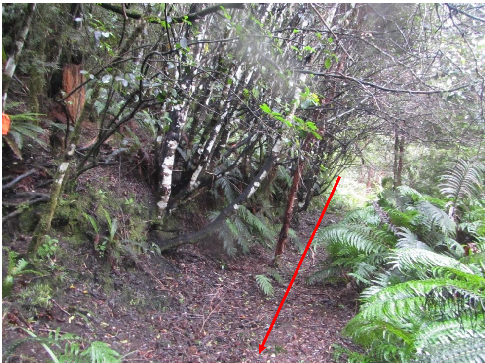
Plate 32: Section 4 of the proposed trail route. A bank alongside the tramline. Red arrow indicates the direction of Ohakune. 16 September 2021.
