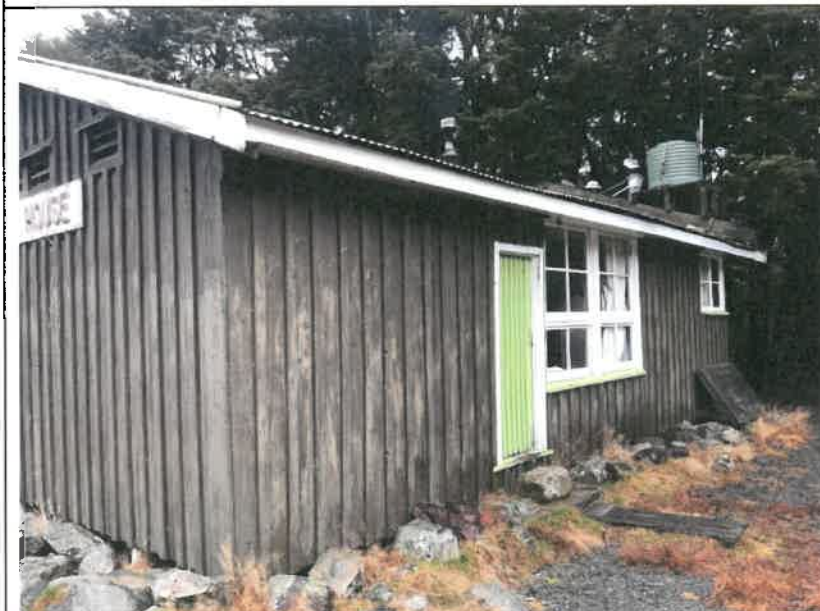
Main Kidson House lodge. Front view from the main clearing. This building is used for cooking etc.
