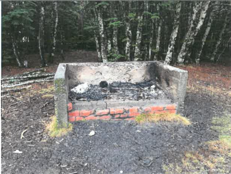
Concrete fireplace at Kidson House.
