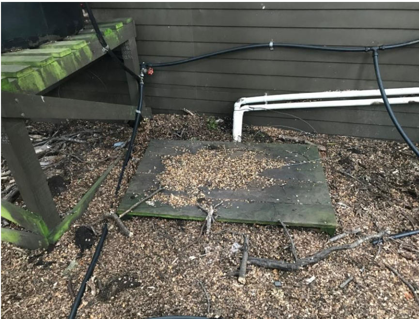
Ground soakage pit next to the washroom
