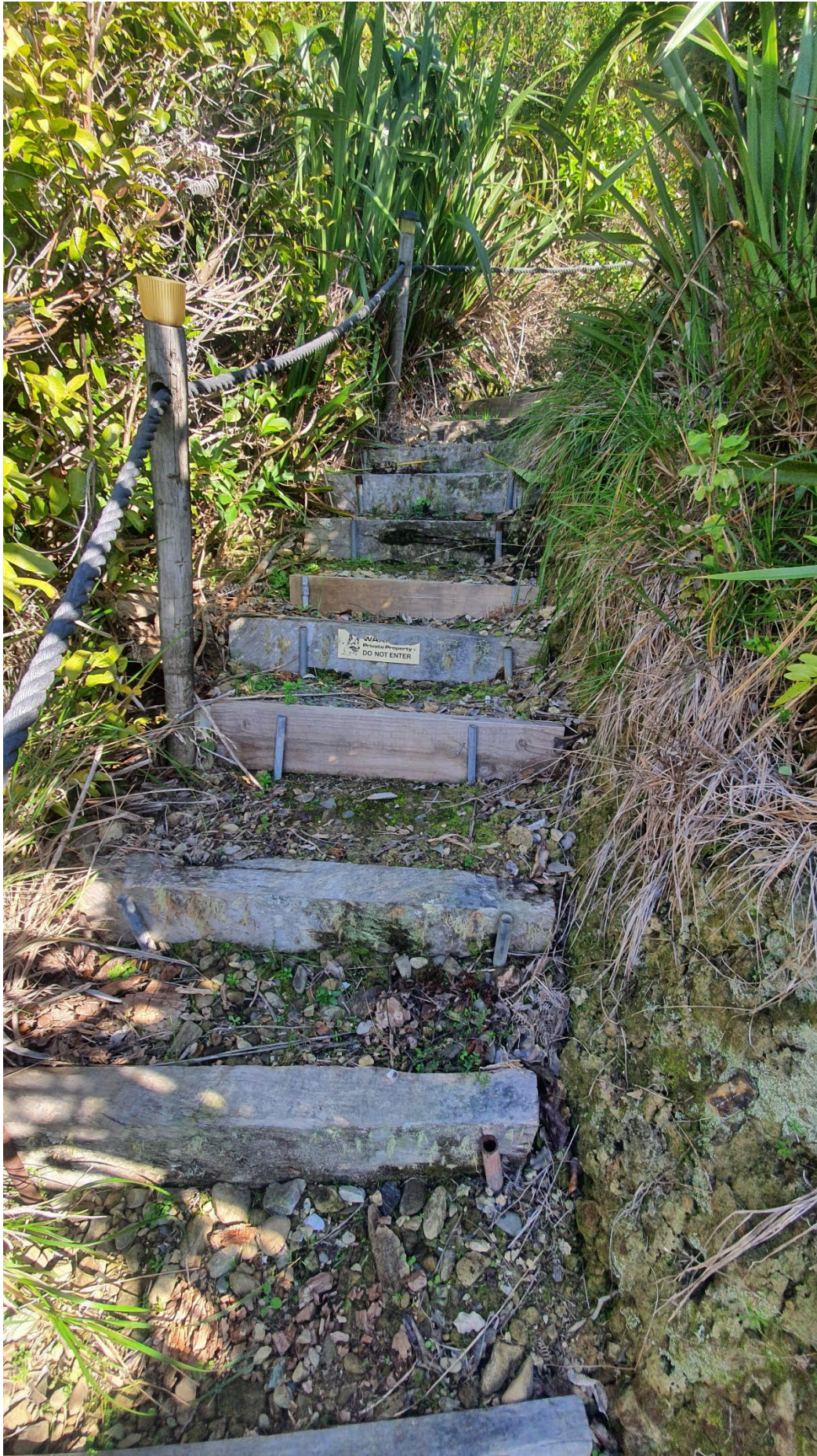
Photos of the structures under the application for McKendry, Paul Francis; King, Gregory John and McKendry, Matthew Leo
